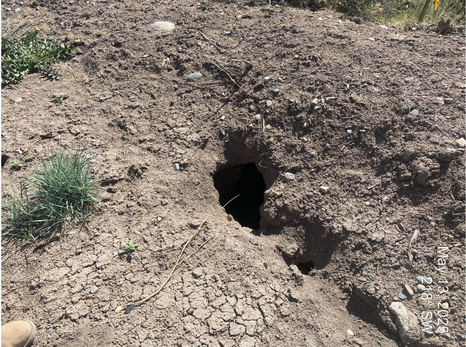
Photo 7. Deep tunnel erosion forming on the western edge perimeter berm.
