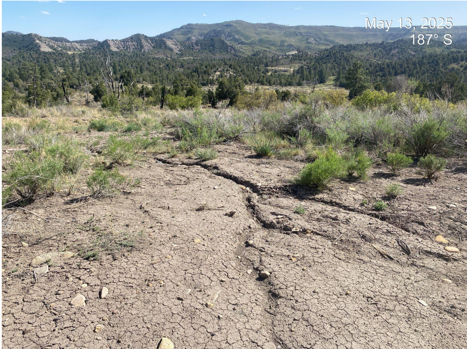
Photo 2. View of erosion issues in the southern portion of the pad facing south.
