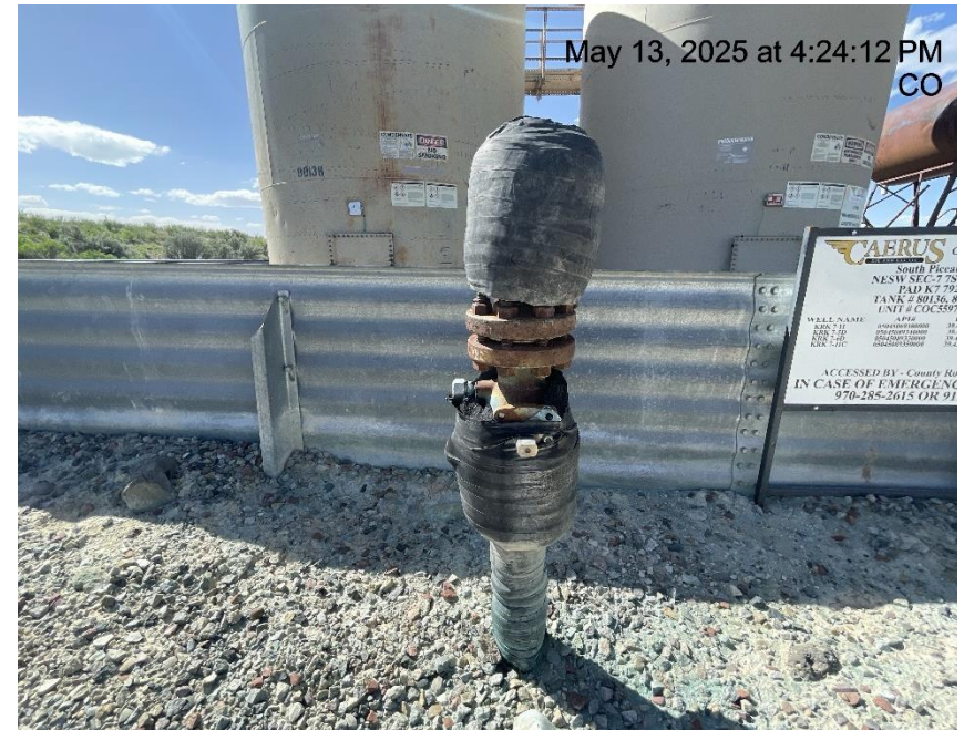
Photo # 822 Unused flowline does not comply with CECMC rules
