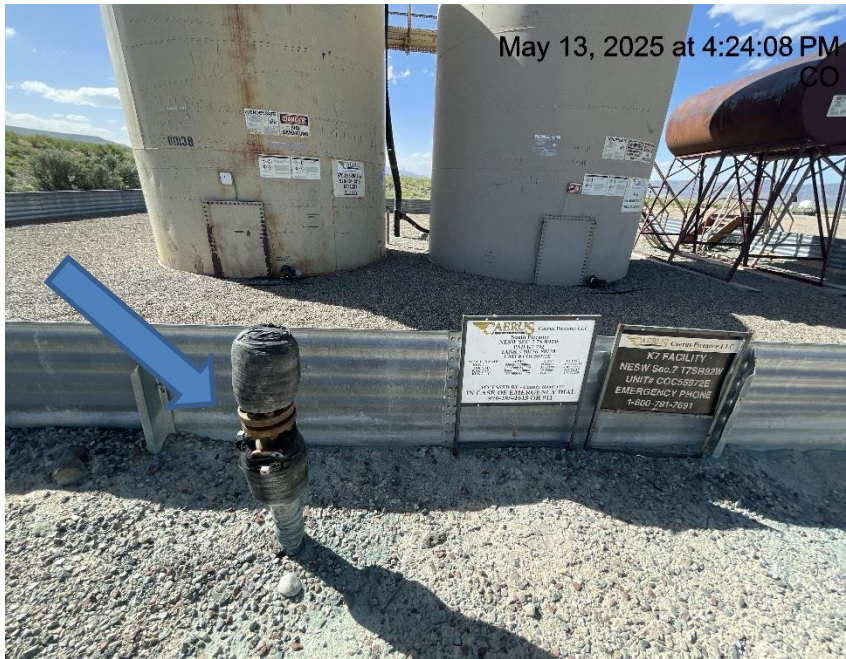
Photo # 821 Unused flowline does not comply with CECMC rules
