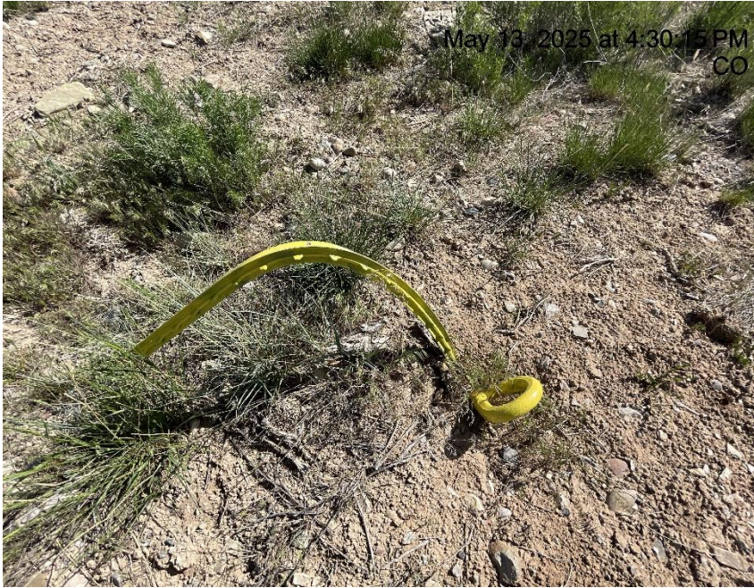
Photo # 825 Improperly marked deadman
