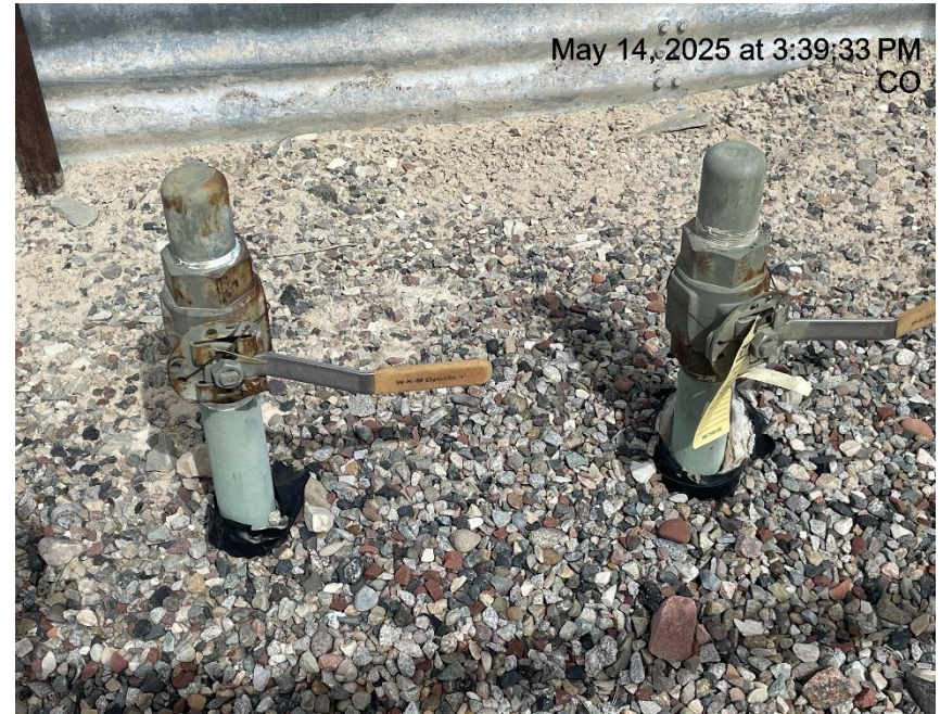
Photo # 1678 Unused flowlines do not comply with CECMC rules
