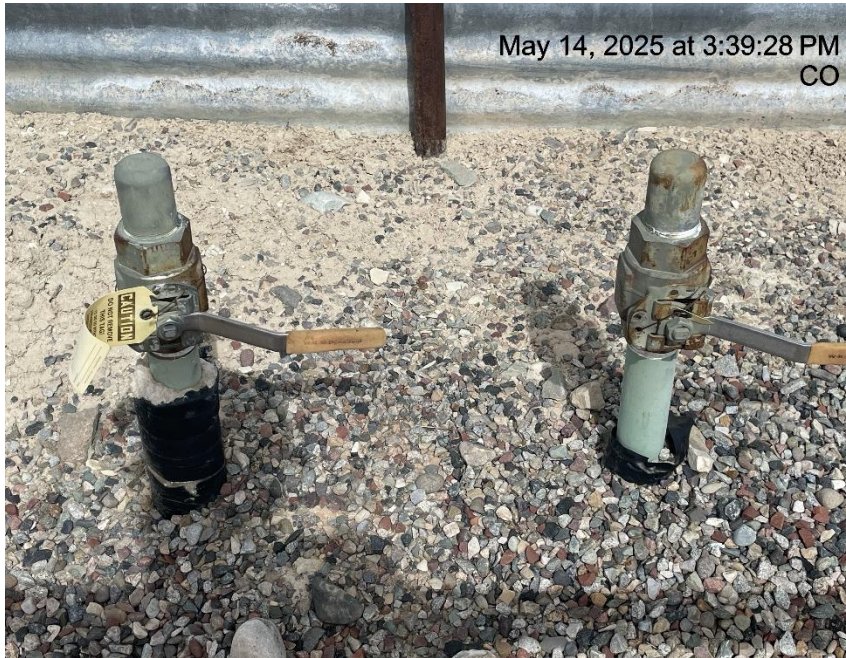
Photo # 1677 Unused flowlines do not comply with CECMC rules
