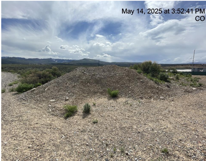
Photo # 1689 Stockpiled soils with no BMP's
