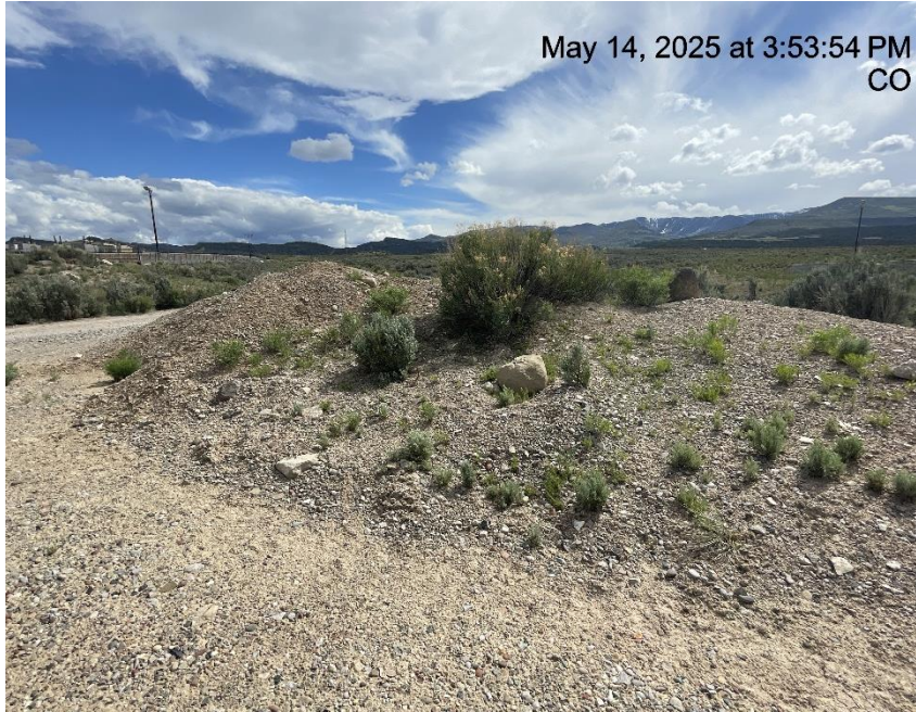
Photo # 1691 Stockpiled soils with no BMP's
