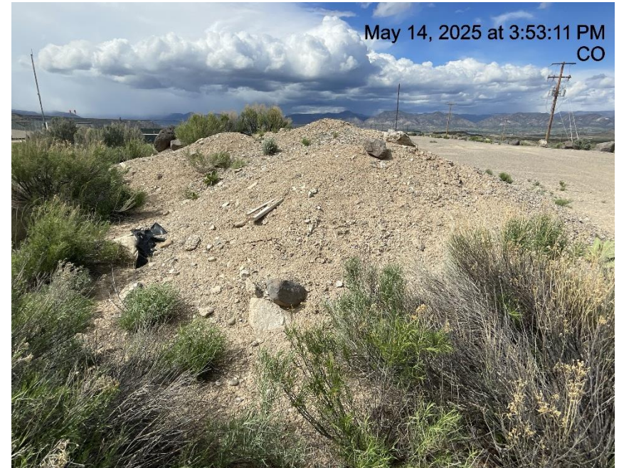
Photo # 1694 Stockpiled soils with no BMP's
