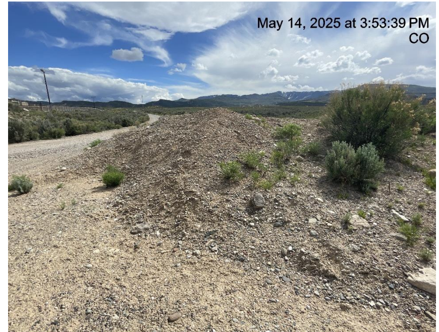
Photo # 1690 Stockpiled soils with no BMP's
