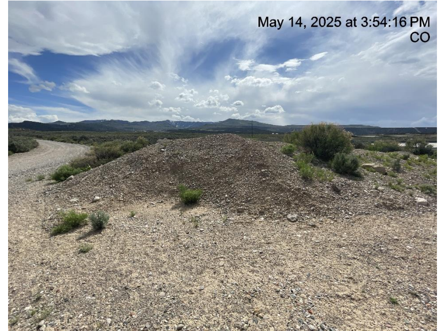
Photo # 1692 Stockpiled soils with no BMP's
