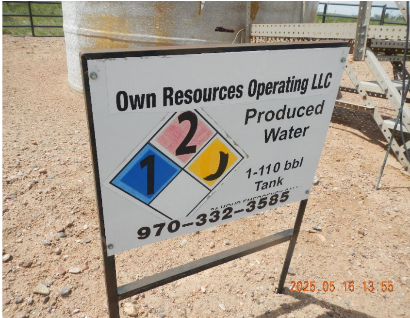
5. Fading Content/Quantity/Hazard sign at produced water tank.
