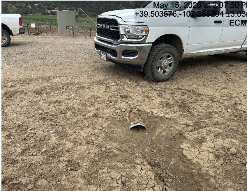
Recent inspection photo of culvert lacks maintained
