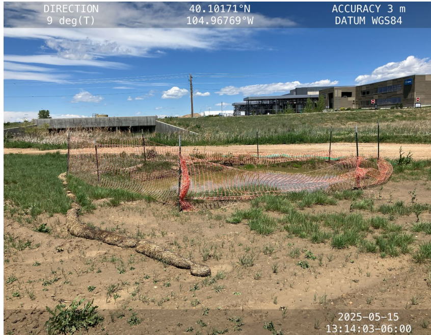
Fencing around the excavation has fallen
