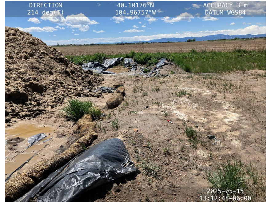
Contaminated soil has overflowed off the line and onto the ground surface
