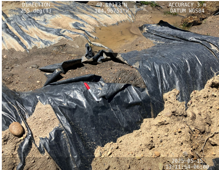
Rips and tears in the liner under the stockpile
