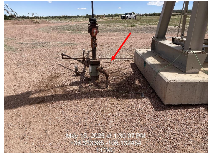
Photo 4 – Stained soils at wellhead
