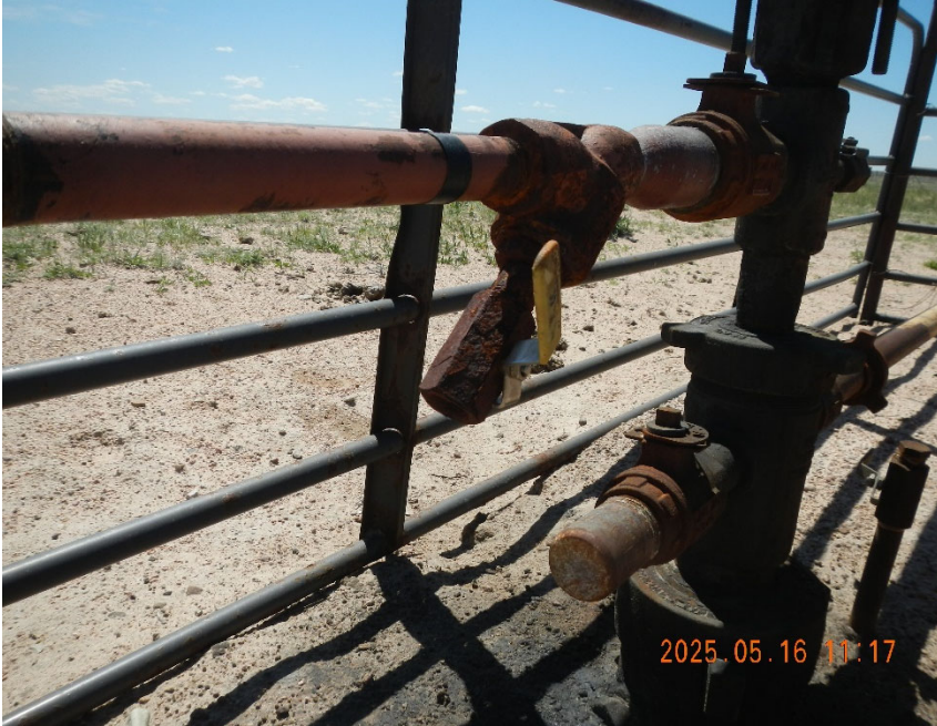
5. Open ended valve on water leg. Note stained soil around Wellhead.
