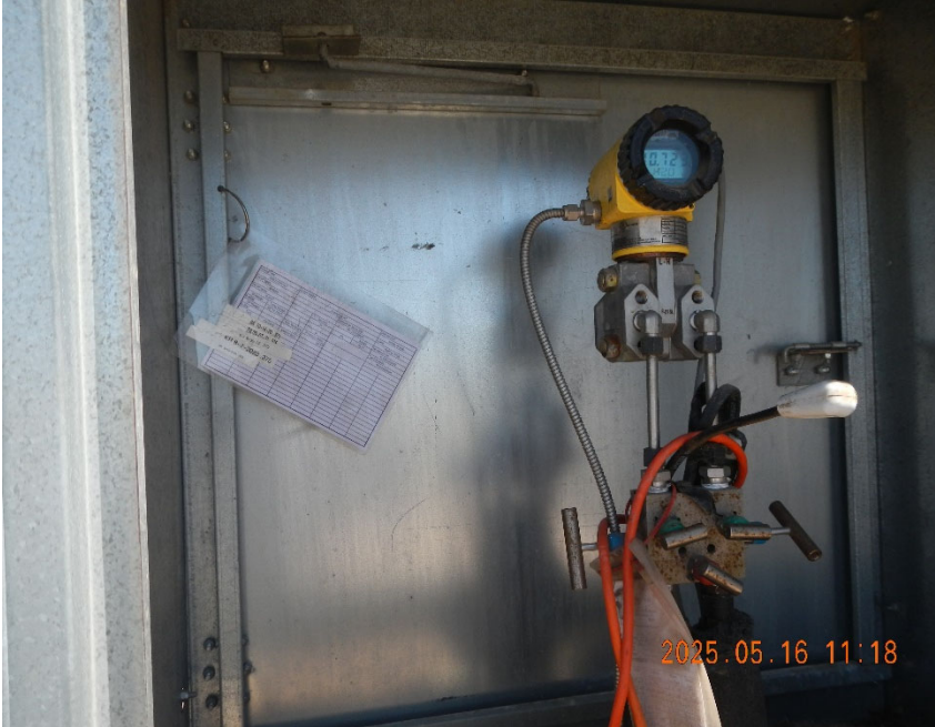
3. Gas Meter inside Meter Box.
