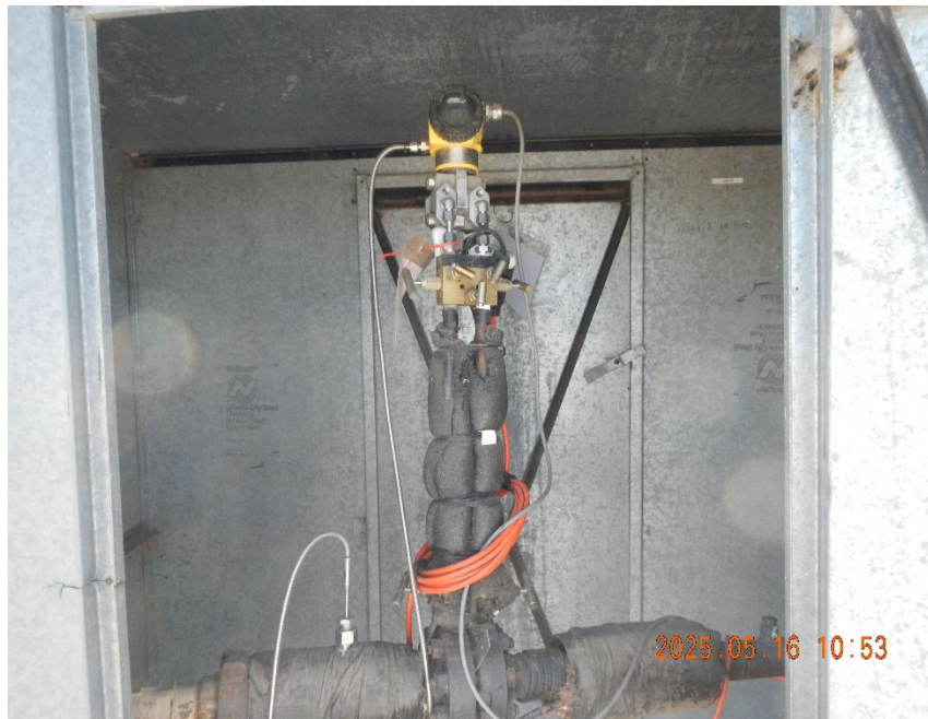
3. Gas Meter inside Meter Shed.
