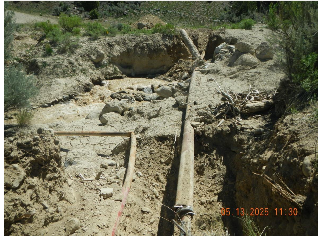
Flowlines excavated to cut out of creek.
