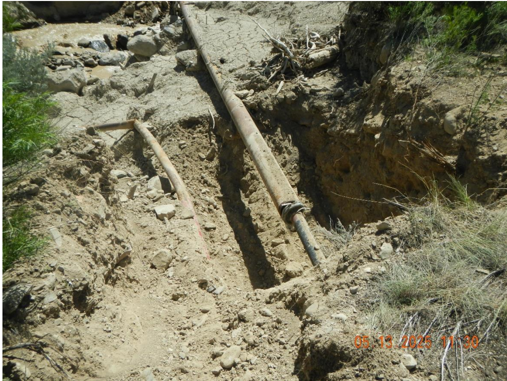
Flowlines excavated to cut out of creek.
