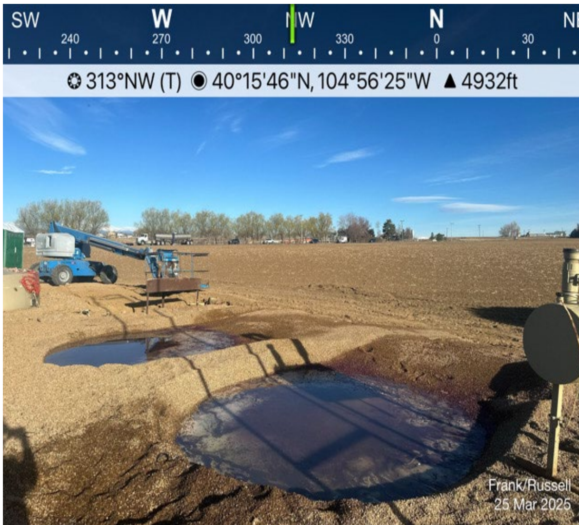
AST01 and AST02 Footprints (exposed tank battery liner at base)
