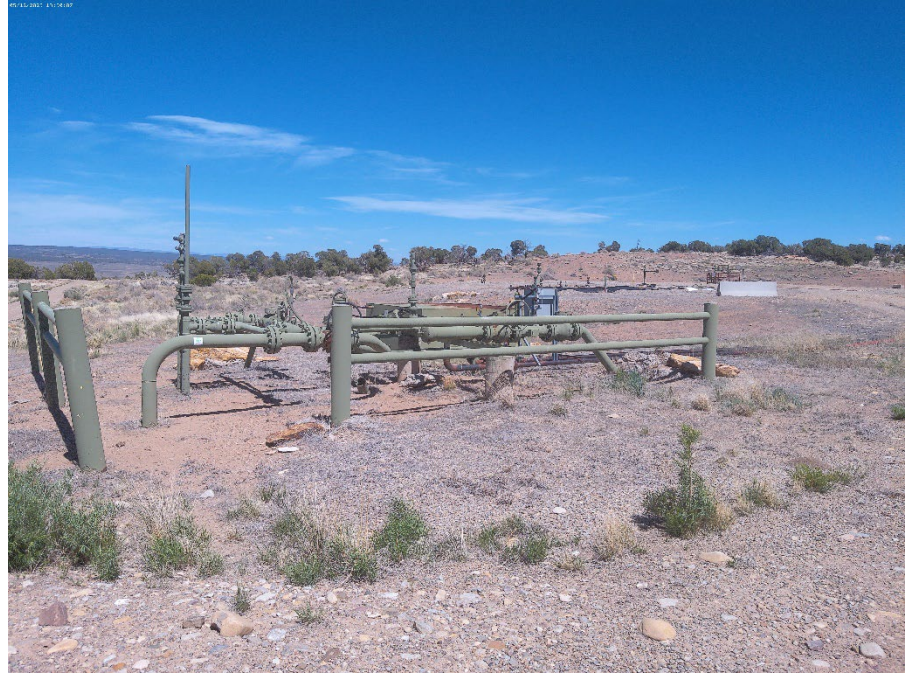
Off location flowlines risers, pig station and blowdown tank
