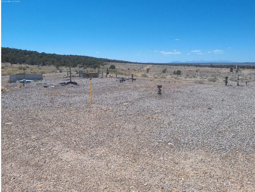
Numerous flowline risers with blind flanges.
