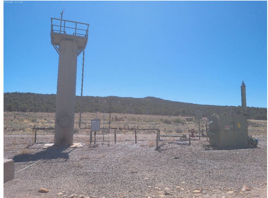
Separator and Dehydrator
