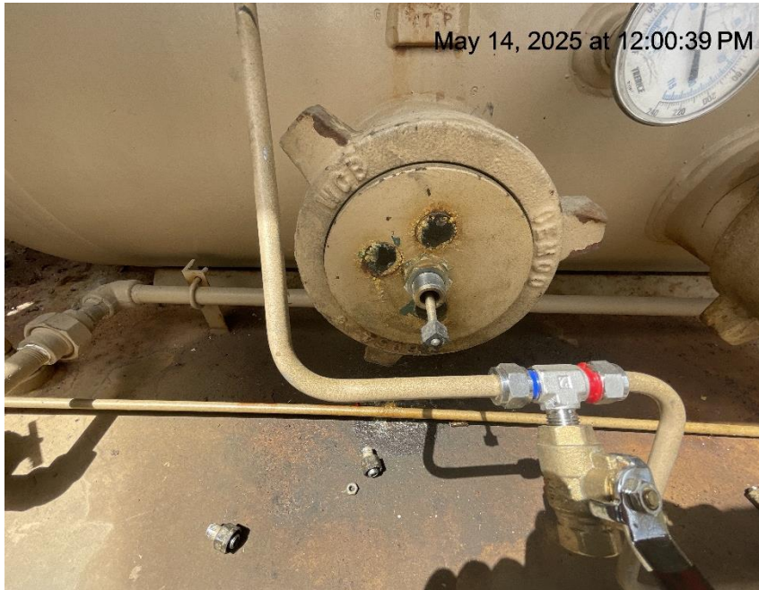
Photo # 913 Water dump controller has been removed from separator unit
