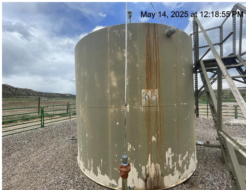
Photo # 905 Staining down side of tank
