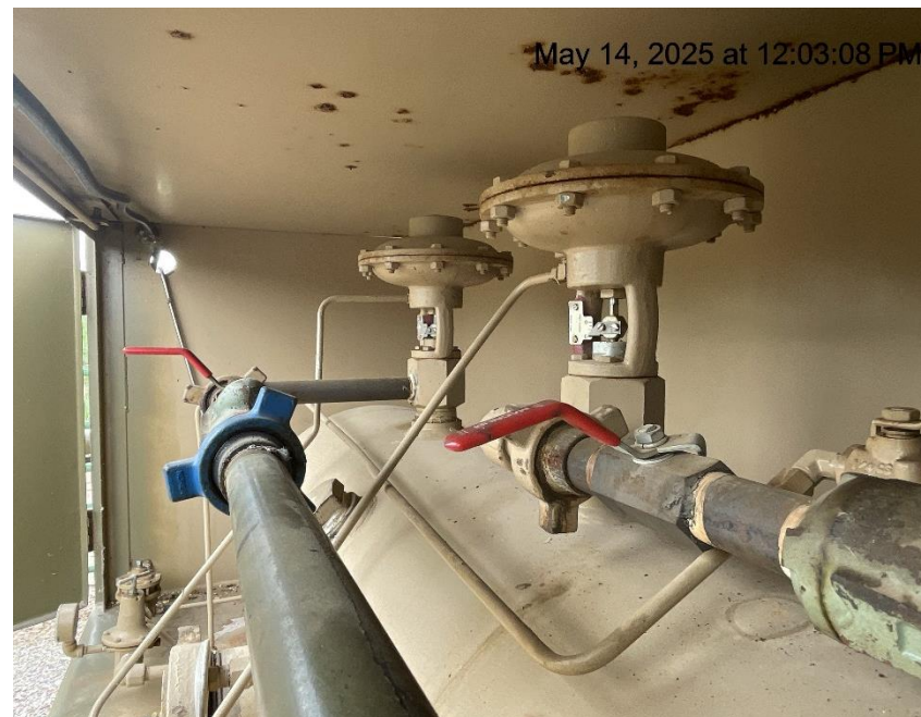
Photo # 906 Valves are shut on water & oil dump lines
