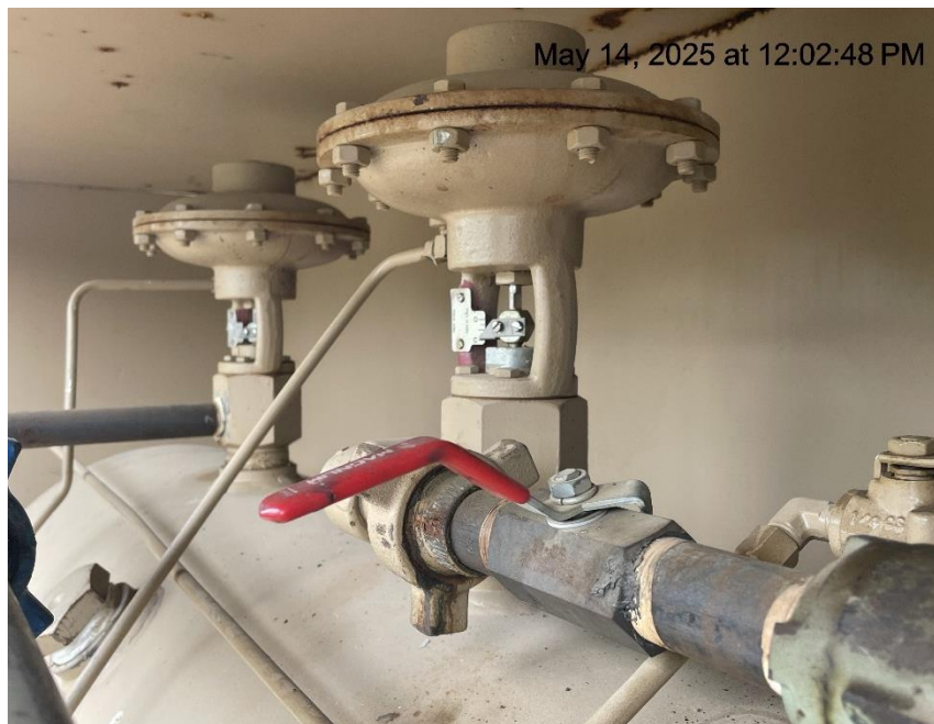
Photo # 909 Valve is shut on oil dump line
