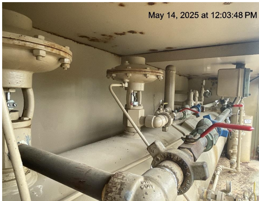
Photo # 911 Valves are shut on water & oil dump lines
