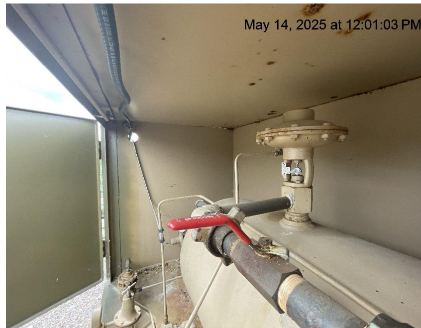
Photo # 910 Valve is shut on water dump line
