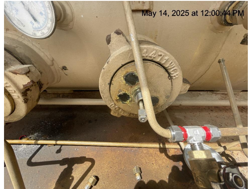
Photo # 914 Oil dump controller has been removed from separator unit
