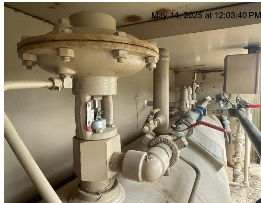
Photo # 908 Valve is shut on oil dump line
