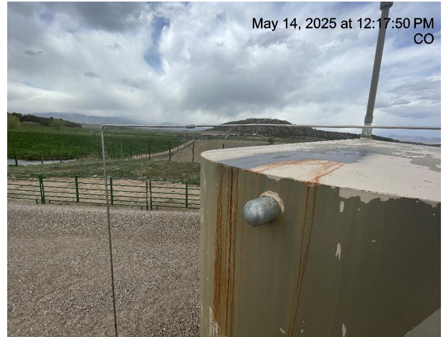
Photo # 904 Staining on top of the tank & down the side of tank that indicates the tank lacks integrity
