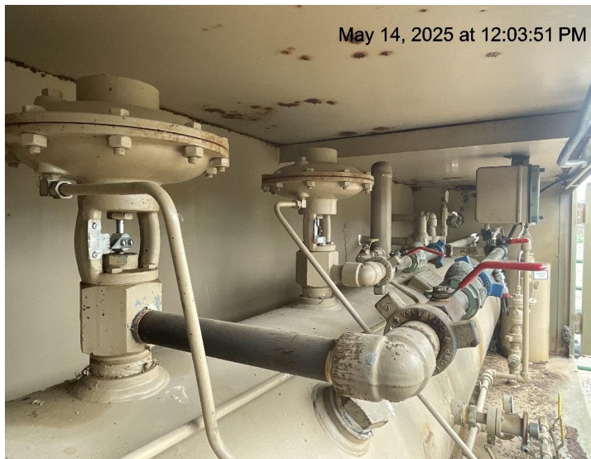
Photo # 907 Valves are shut on water & oil dump lines
