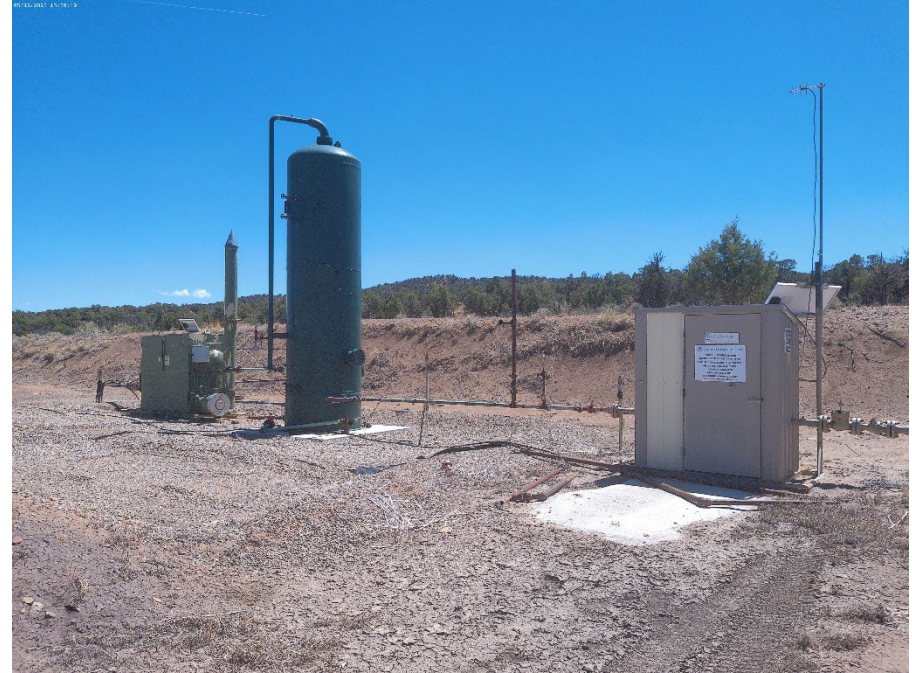
Separator, Dehydrator and Meter housing
