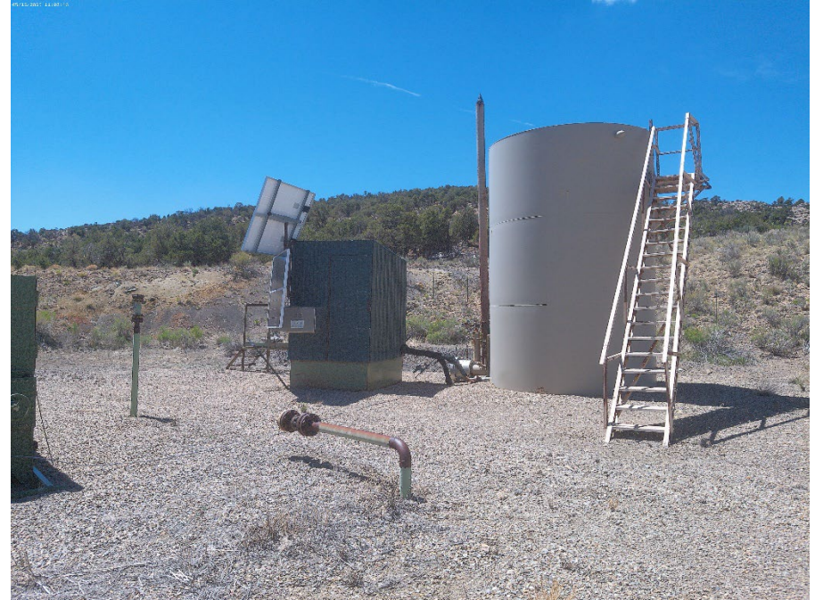
Fresh water tanks
