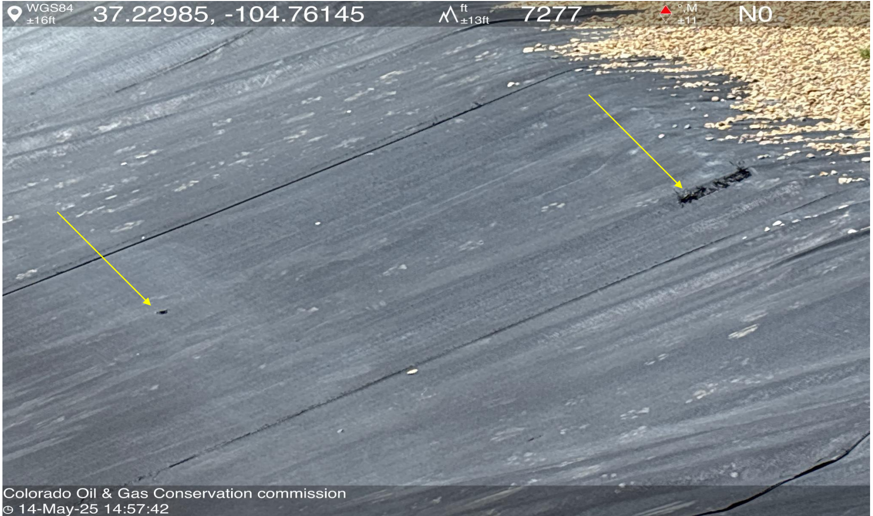
PHOTO 5: TWO SMALL HOLES IN PIT LINER ( HOLE IN LINER IS WELL ABOVE FLUID LEVEL IN PIT). Contact COGCC EPS staff for directives. CA DATE 5/16/2024
