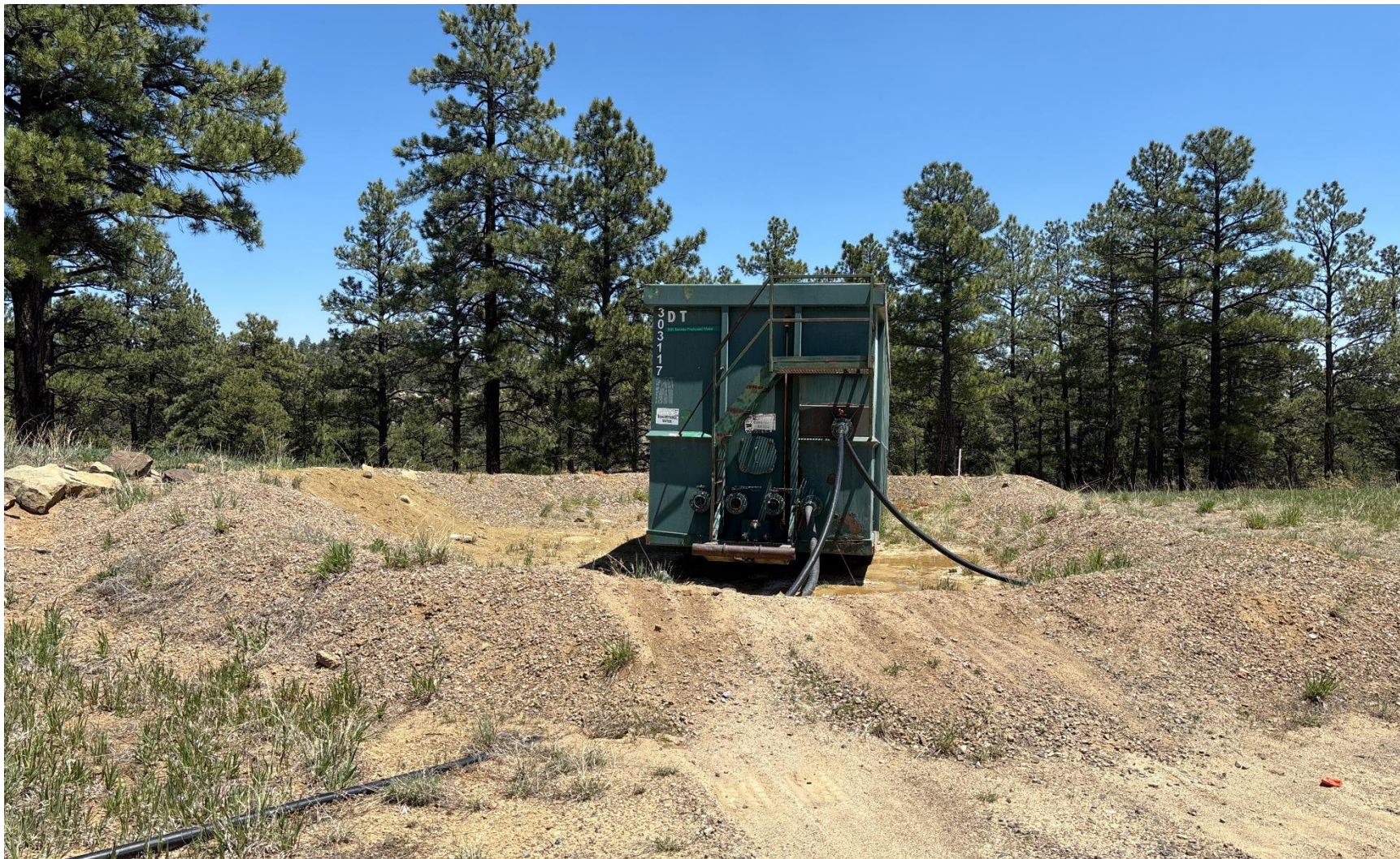
PHOTO 5: PRODUCED WATER TANK BATTERY. NO NFPA STICKER ON TANK BATTERY. Install sign to comply with Rule 605.h. THIS IS THE SECOND NOTICE FOR THIS CA, IMMEDIATE ACTION IS REQUIRED.
