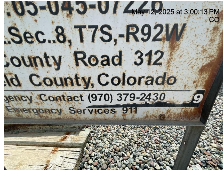
Photo # 479 Emergency contact # on wellhead sign incorrect/not in compliance with CECMC rules
