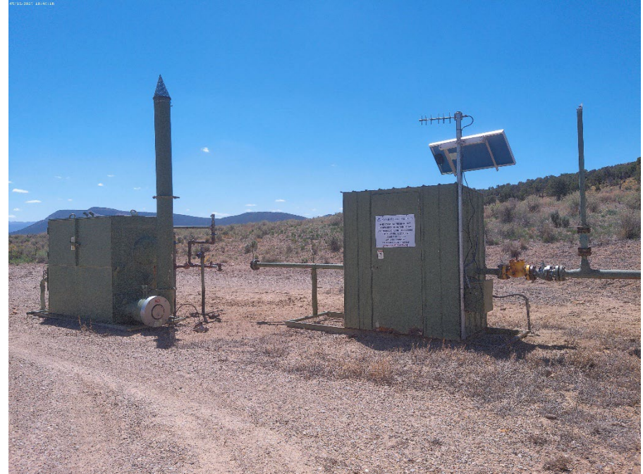
Separator and Meter housing
