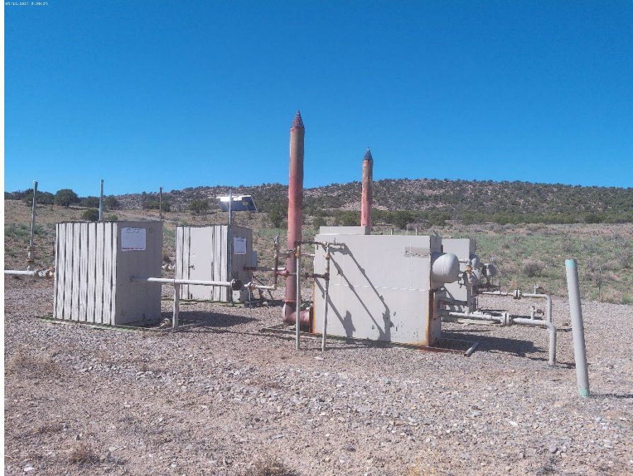
Separators and Meter housings
