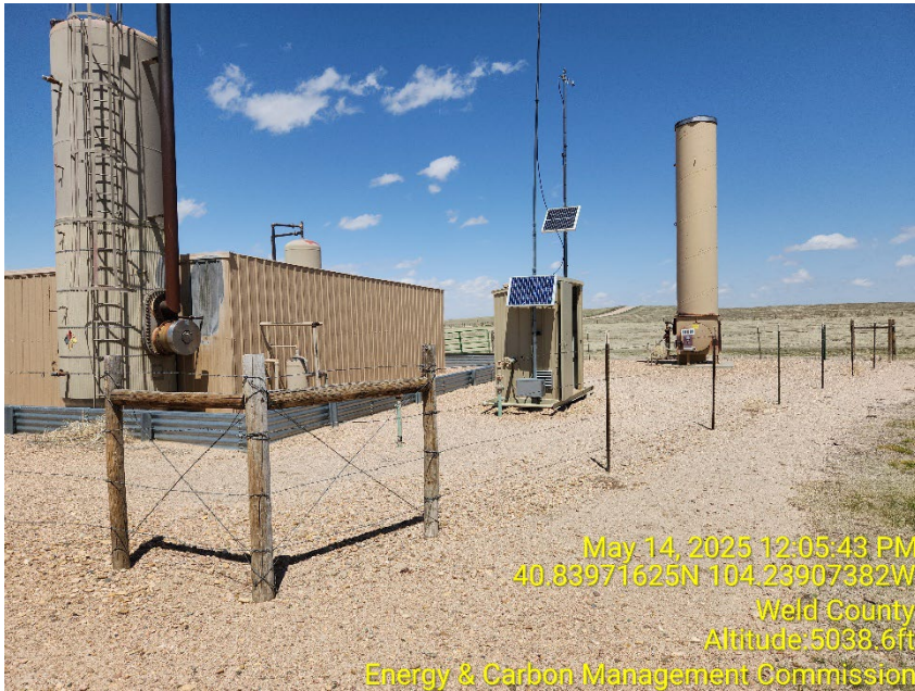
Photo 7 – Heater Treater, Gas Meter and ECD
