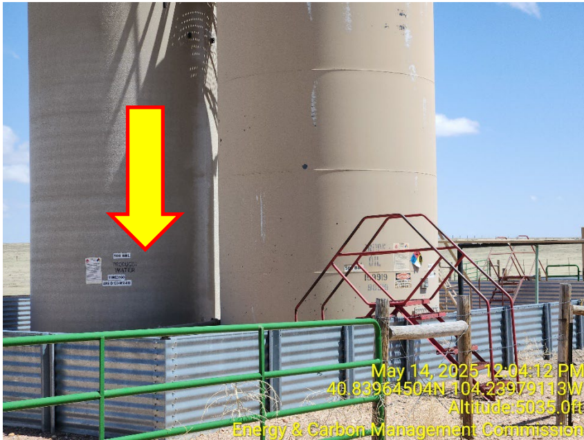
Photo 3 – NFPA Label missing on Water Tank
