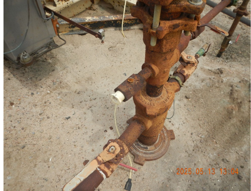
4. Open ended line noted in previous FIR. CA completed and plug installed on tubing line.
