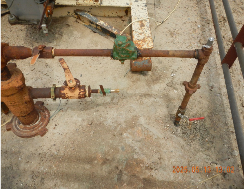
3. View where previous FIR had noted release from check valve. CA completed with no fluid release at check valve.
