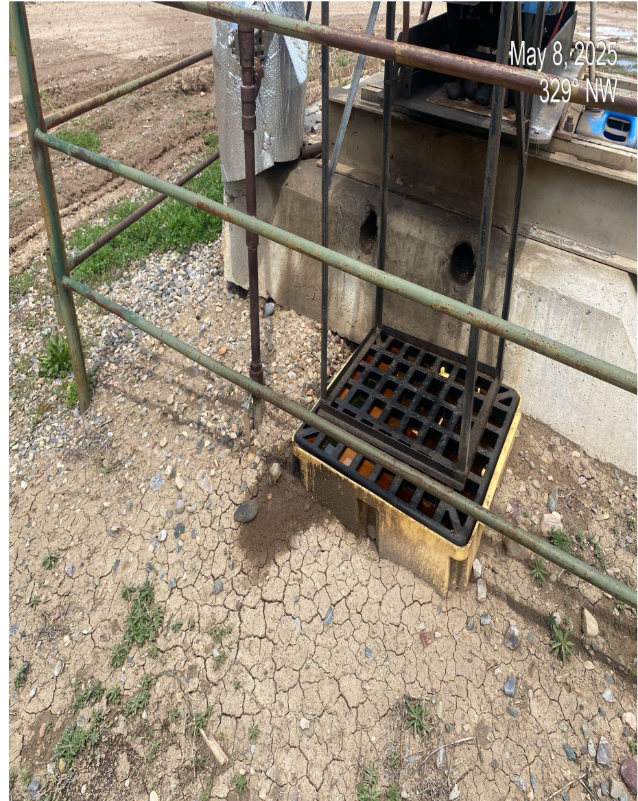
Photo 3. Stained soils at lube tank secondary contaminants.
