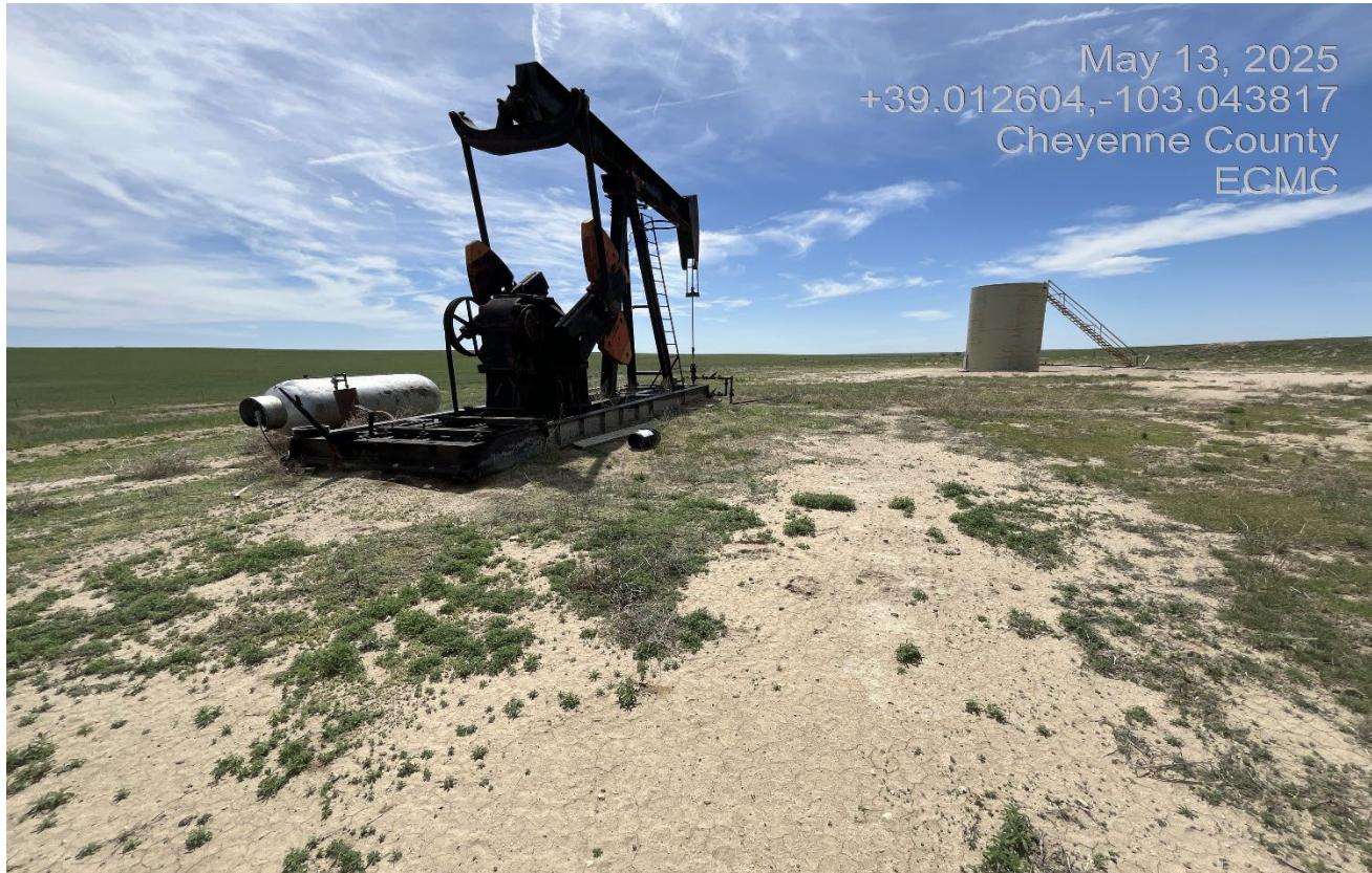
Photo 2. Facing toward the wellhead pumpjack.
