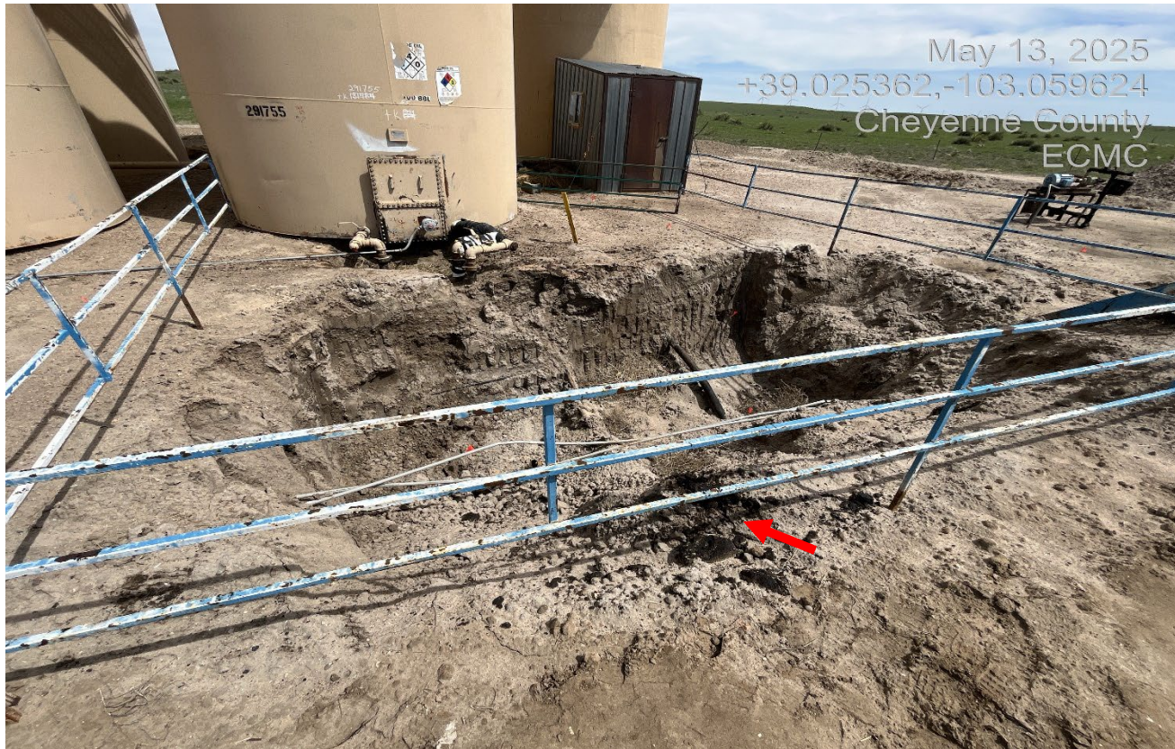
Photo 2. There is an active remediation occurring at the battery. It appears there are still impact shown at red arrow that should be cleaned up better..
