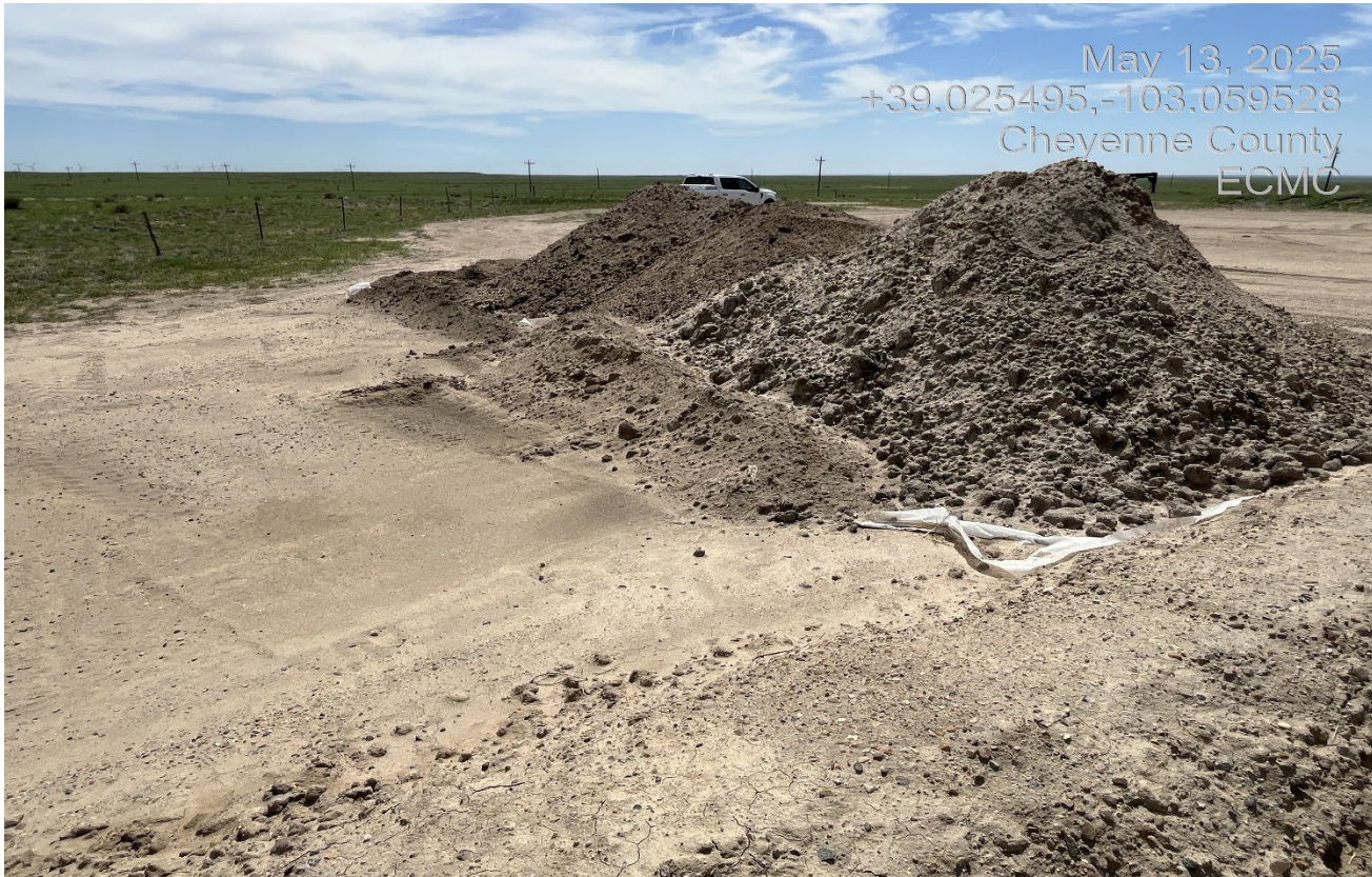
Photo 4. Facing toward the impact material stored onsite. A secondary containment berm needs to be installed around the entire pile.
