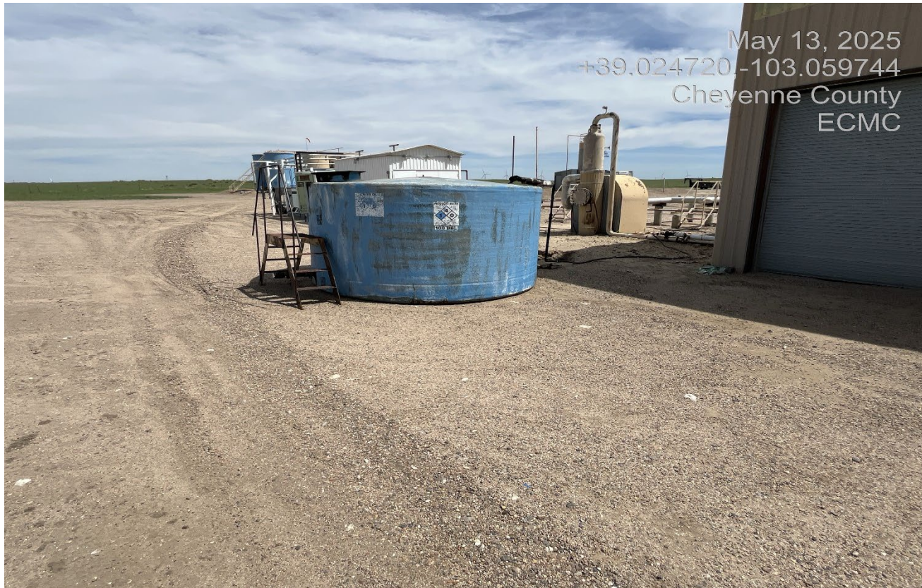
Photo 8. This active tank has no secondary containment.
