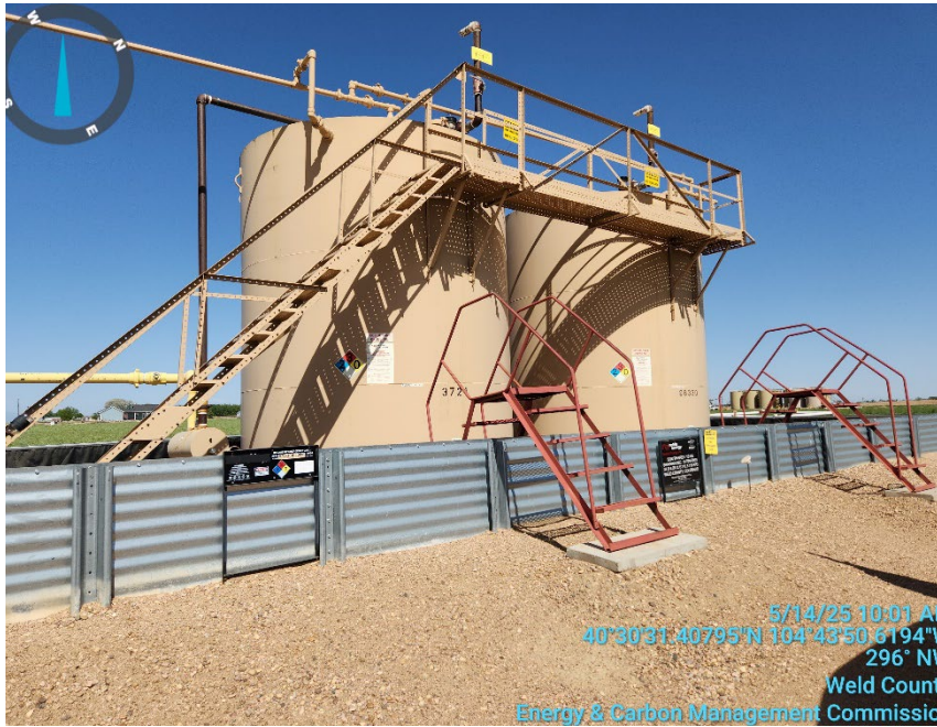
Photo 5: tank battery
