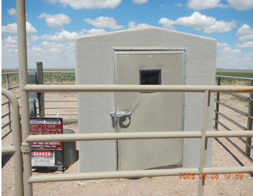
5. View of Well House.
