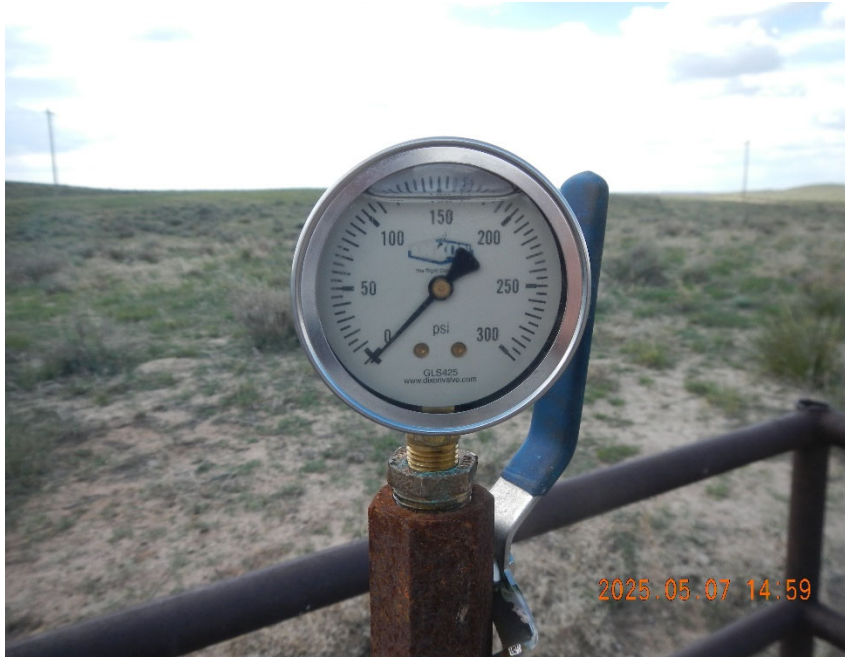
3. Pressure gauge installed on tubing valve.
