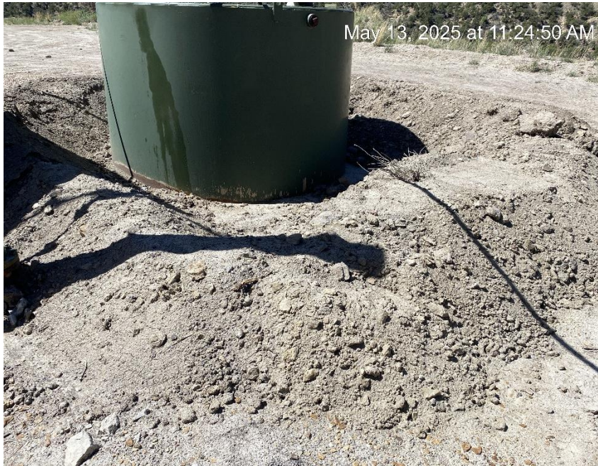
Tank berm capacity inadequate
