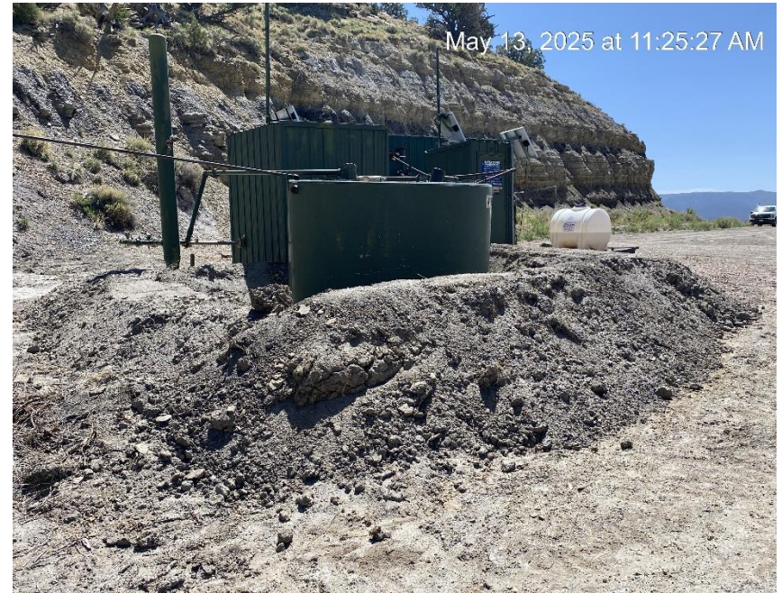
Tank berm capacity inadequate
