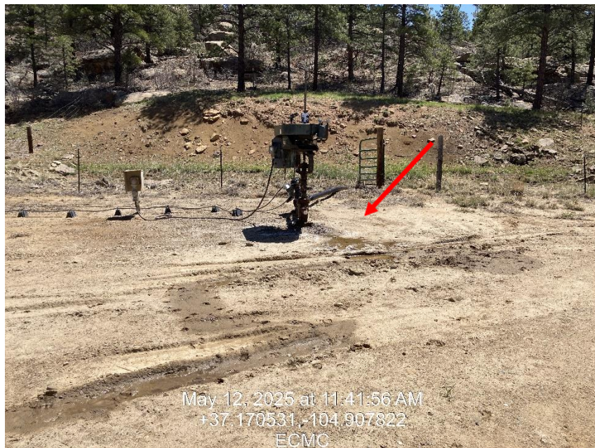
Photo 3 – V wellhead, leaking packing
