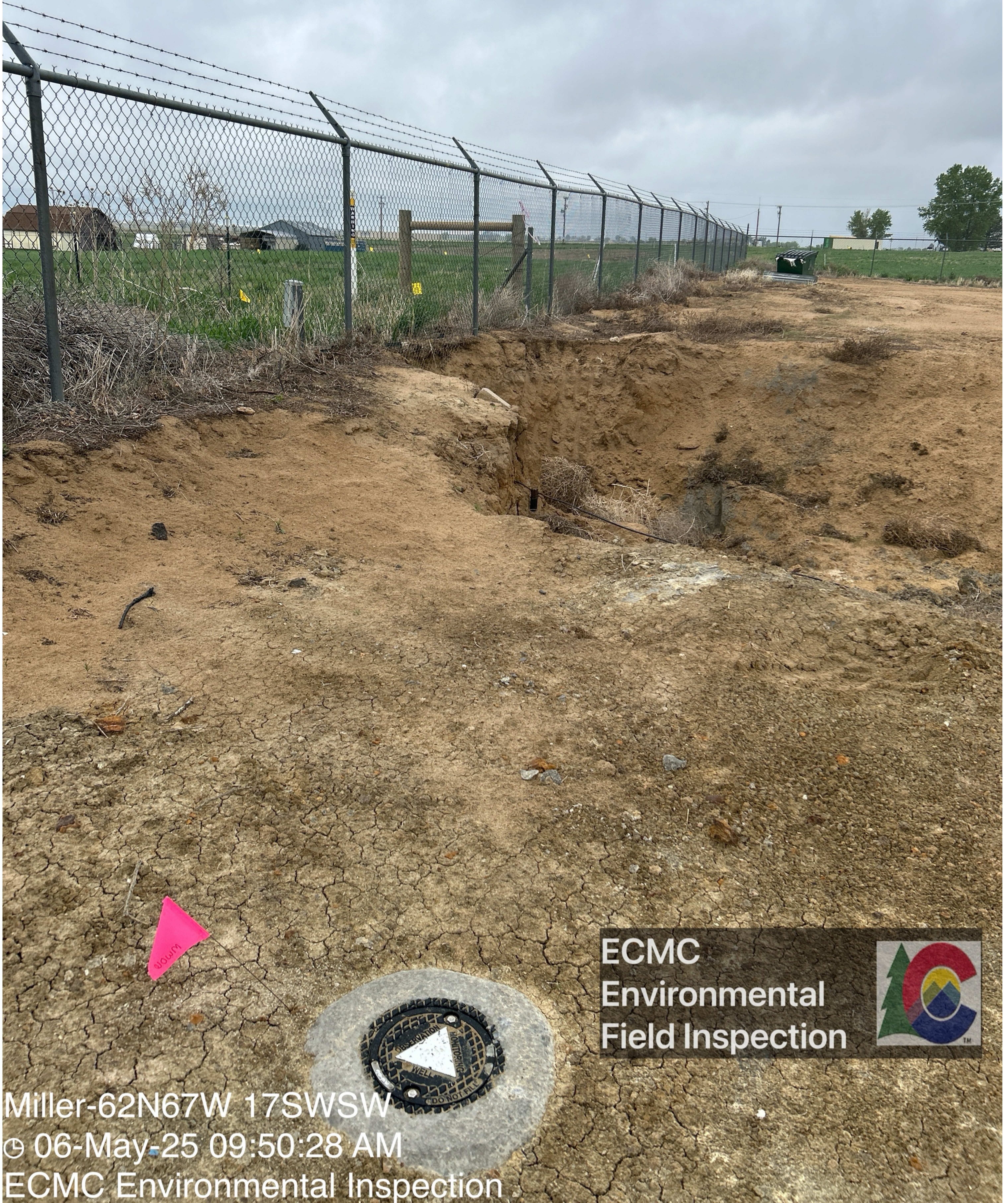
A monitoring well completed as a flush mount was observed adjacent to the excavation.
