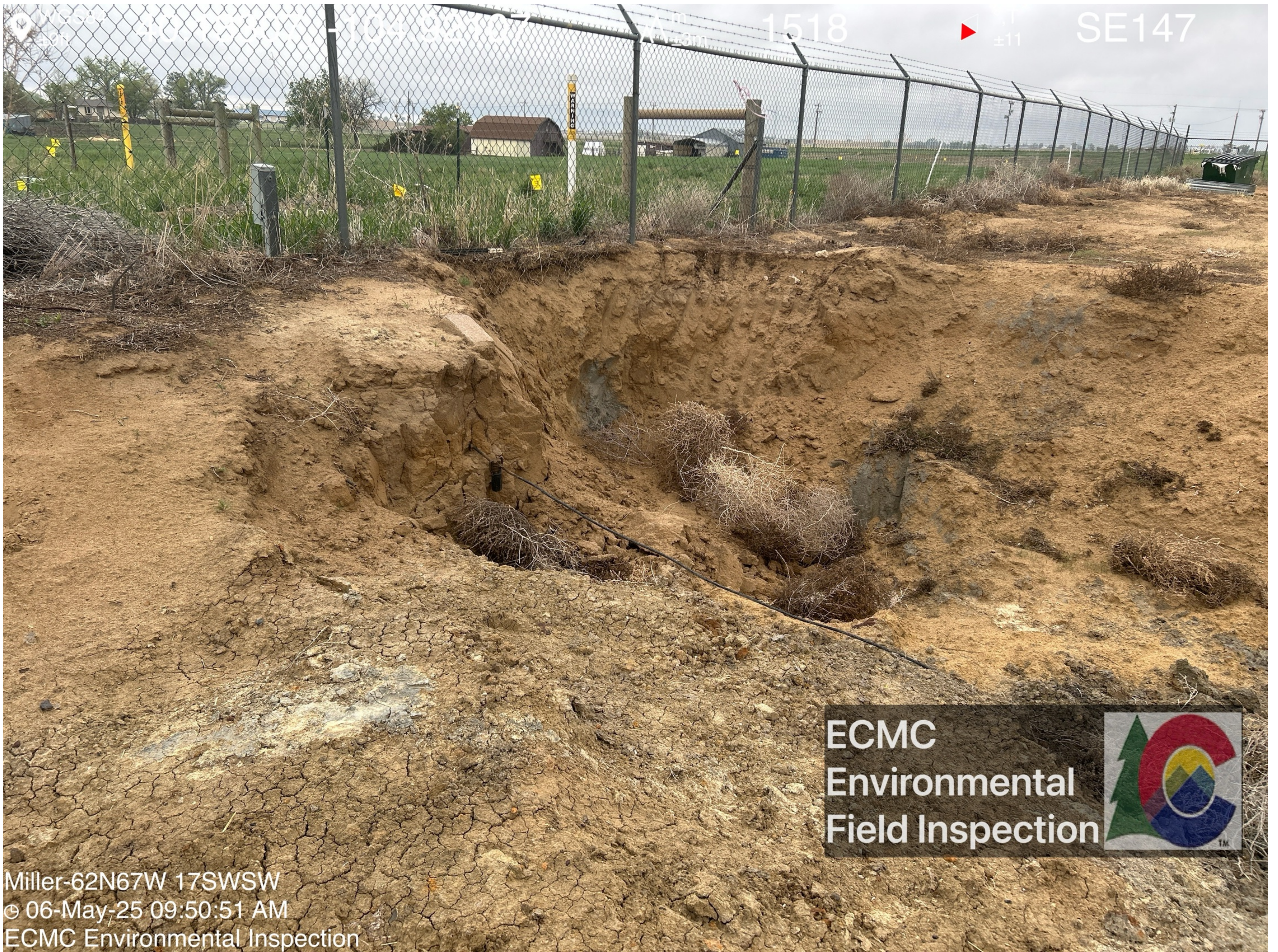
Gray staining is visible on the sidewalls of the excavation. A black wire extends along the excavation.
