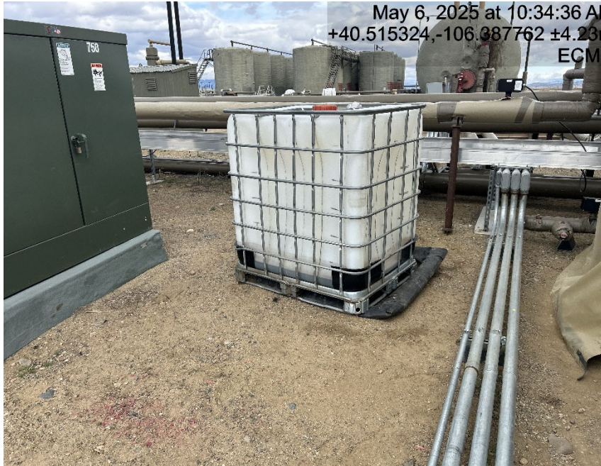
Containment insufficient
