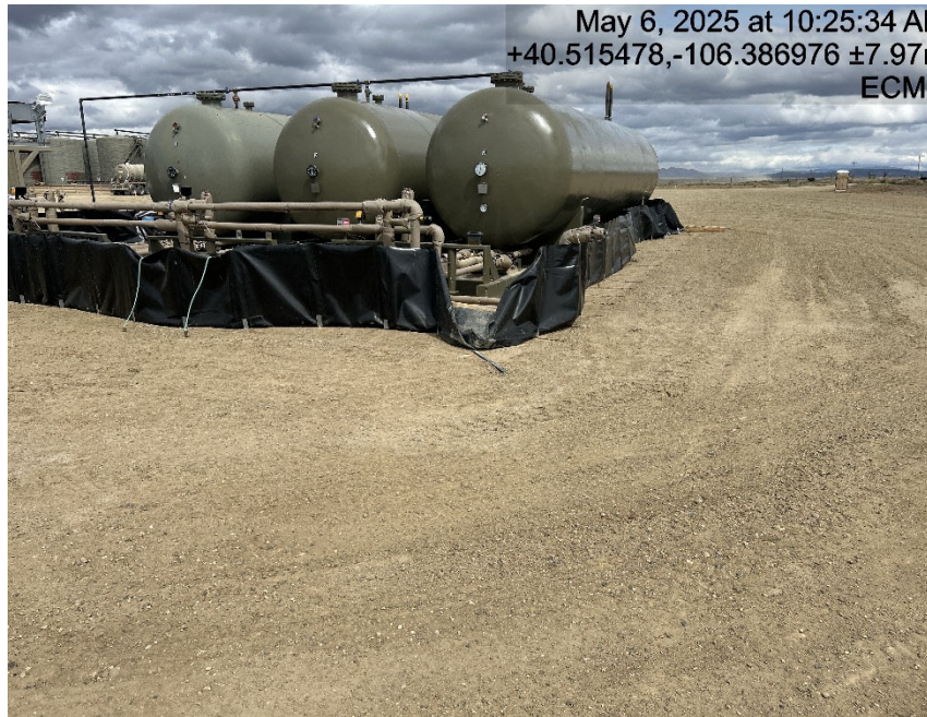
Stored equipment and containment failing
