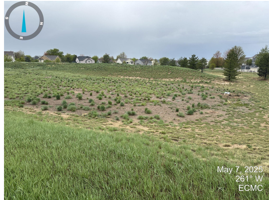
Photo 4. Looking west across the south side of the tank battery location. Illustrating lower vegetation establishment and bare areas.
