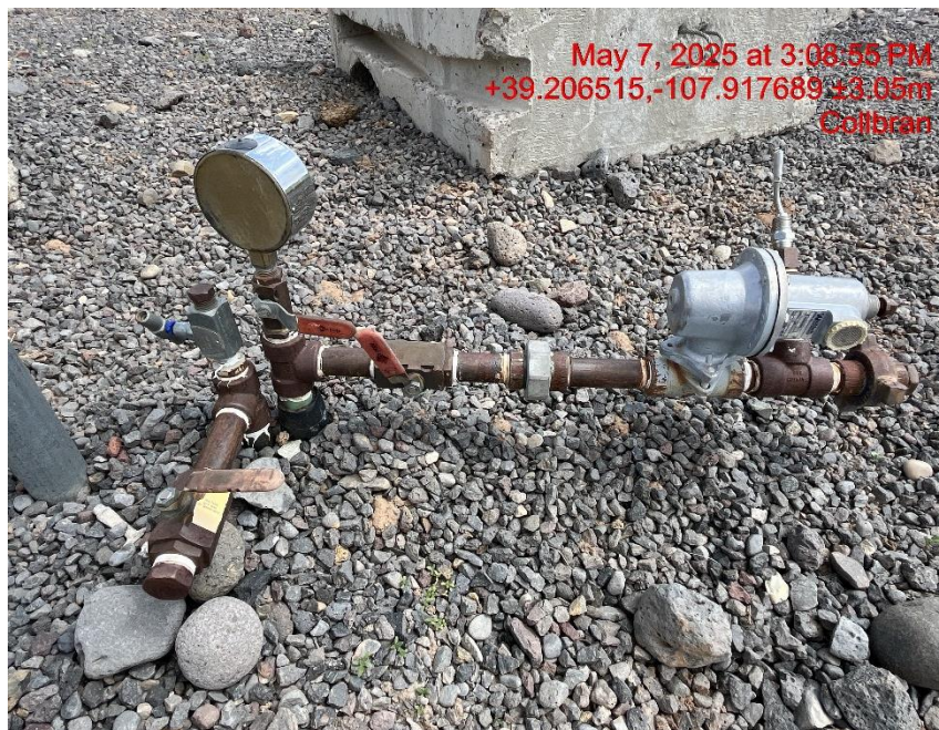
Photo # 7199 Unused flowlines near pump house lack lockout tagout (OOSLAT)
