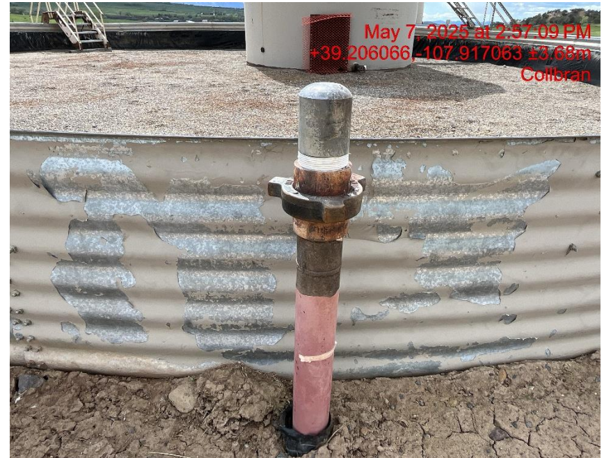
Photo # 7183 Unused flowline at tank battery lacks lockout tagout (OOSLAT)
