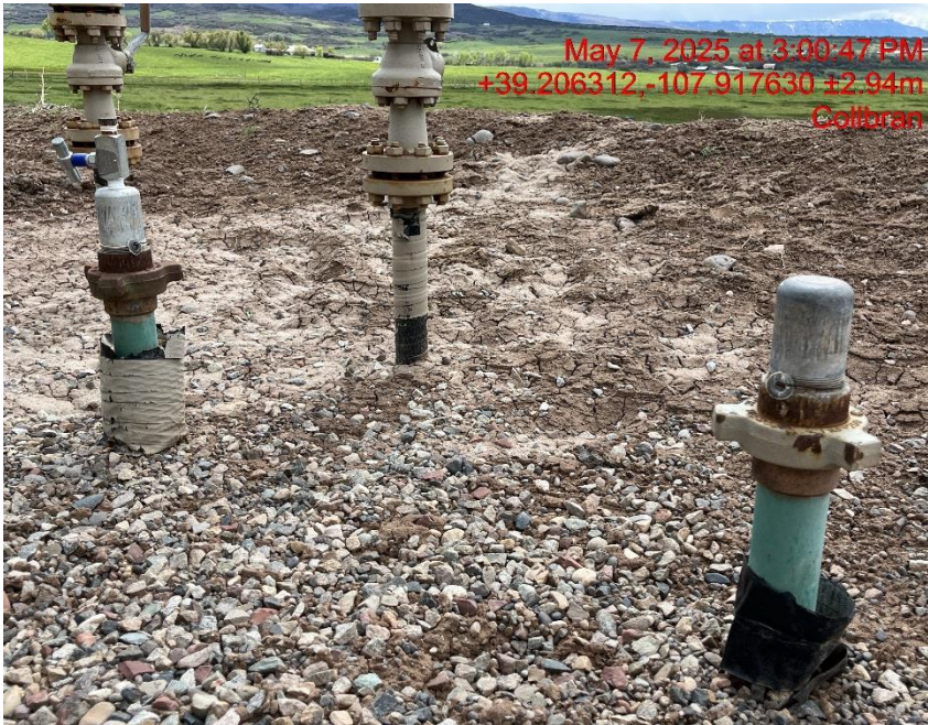
Photo # 7189 Unused flowlines at separators lack lockout tagout (OOSLAT)
