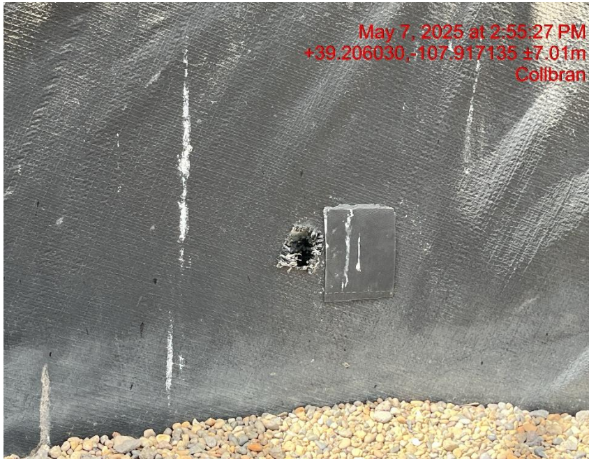
Photo # 7179 Multiple holes in both secondary containments on location liners/liners need maintenance
