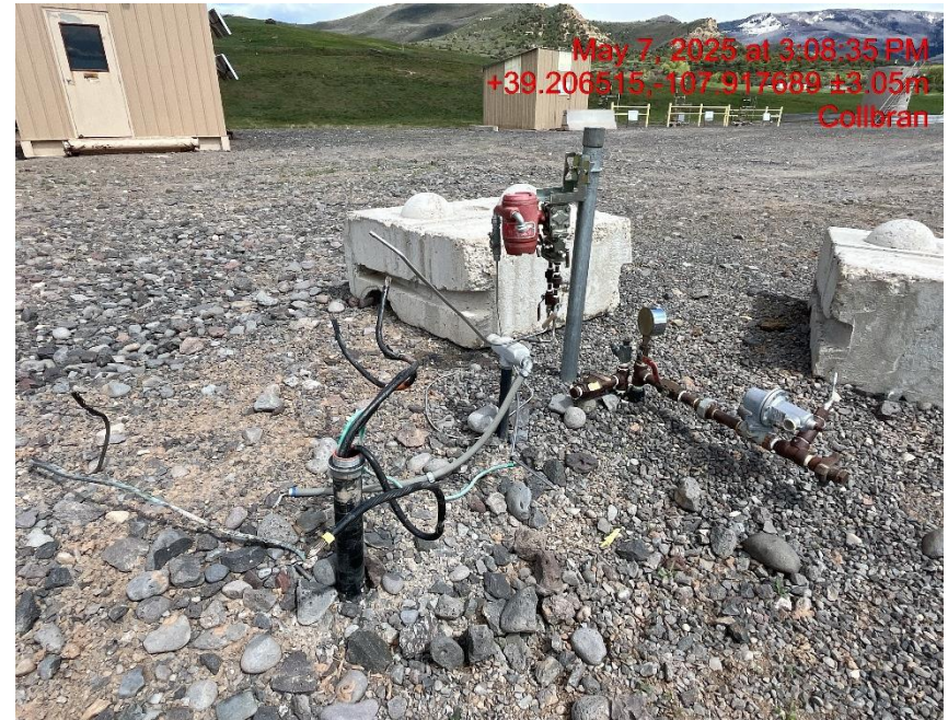
Photo # 7197 Unused flowlines near pump house lack lockout tagout (OOSLAT)
