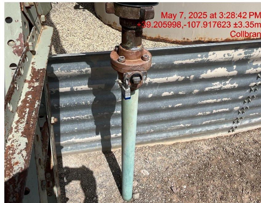
Photo # 7223 Unused flowline at tank battery lacks lockout tagout (OOSLAT)
