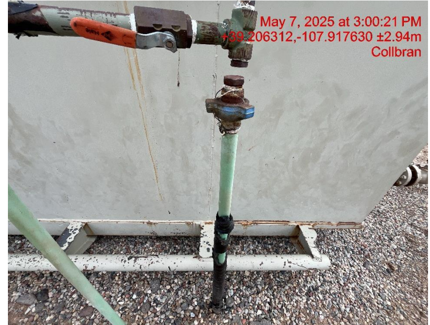
Photo # 7188 Unused flowline at separators lack lockout tagout (OOSLAT)
