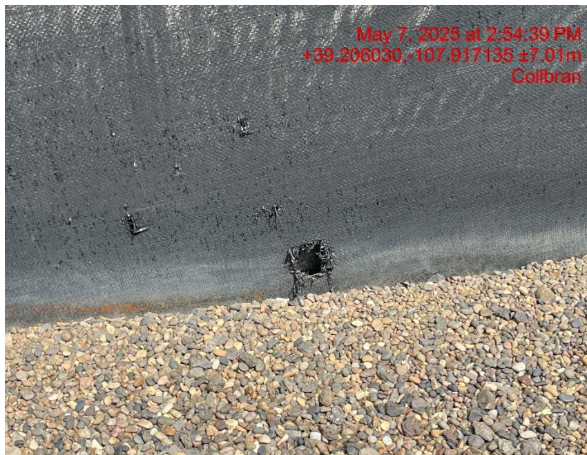
Photo # 7175 Multiple holes in both secondary containments on location liners/liners need maintenance
