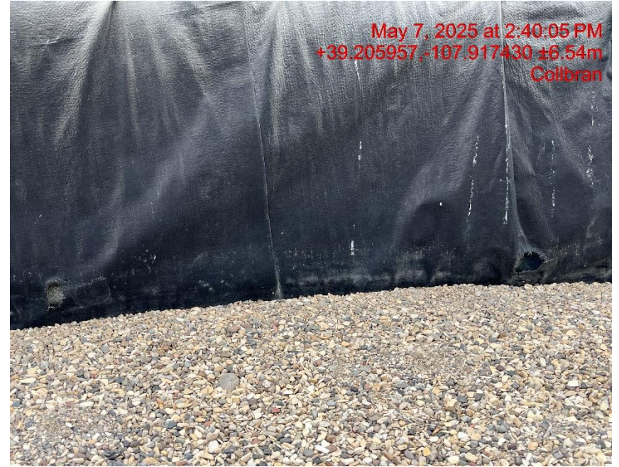
Photo # 7153 Multiple holes in both secondary containments on location liners/liners need maintenance
