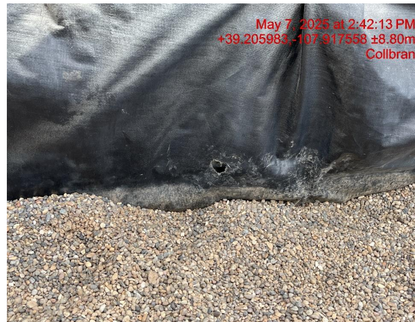
Photo # 7156 Multiple holes in both secondary containments on location liners/liners need maintenance
