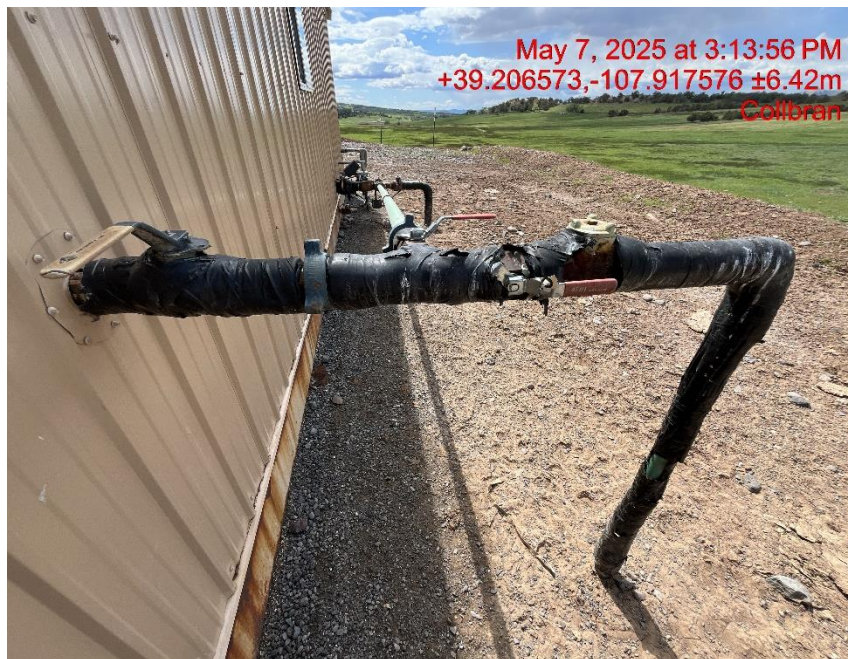
Photo # 7208 Unused flowlines at pump house lack lockout tagout (OOSLAT)
