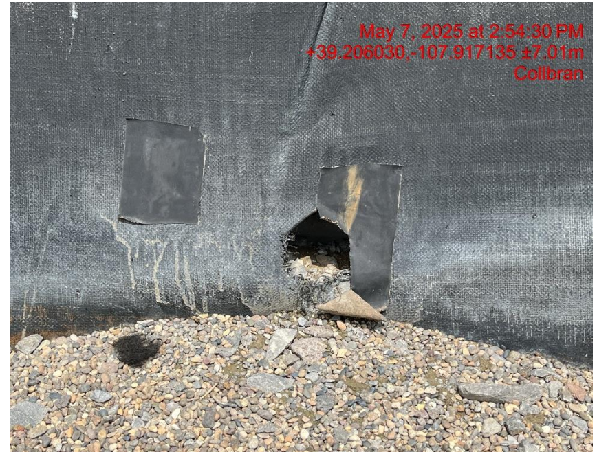
Photo # 7174 Multiple holes in both secondary containments on location liners/liners need maintenance
