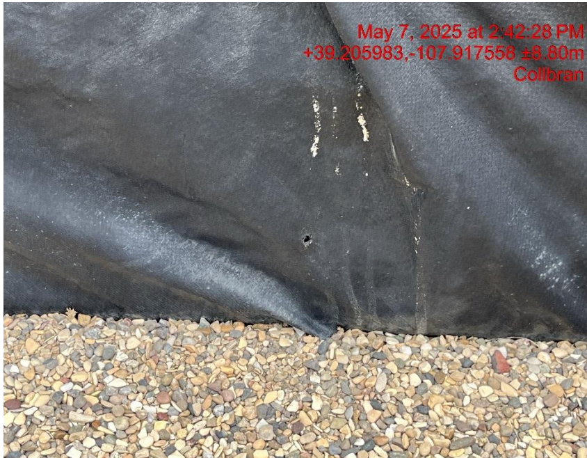
Photo # 7157 Multiple holes in both secondary containments on location liners/liners need maintenance
