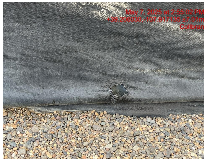
Photo # 7176 Multiple holes in both secondary containments on location liners/liners need maintenance
