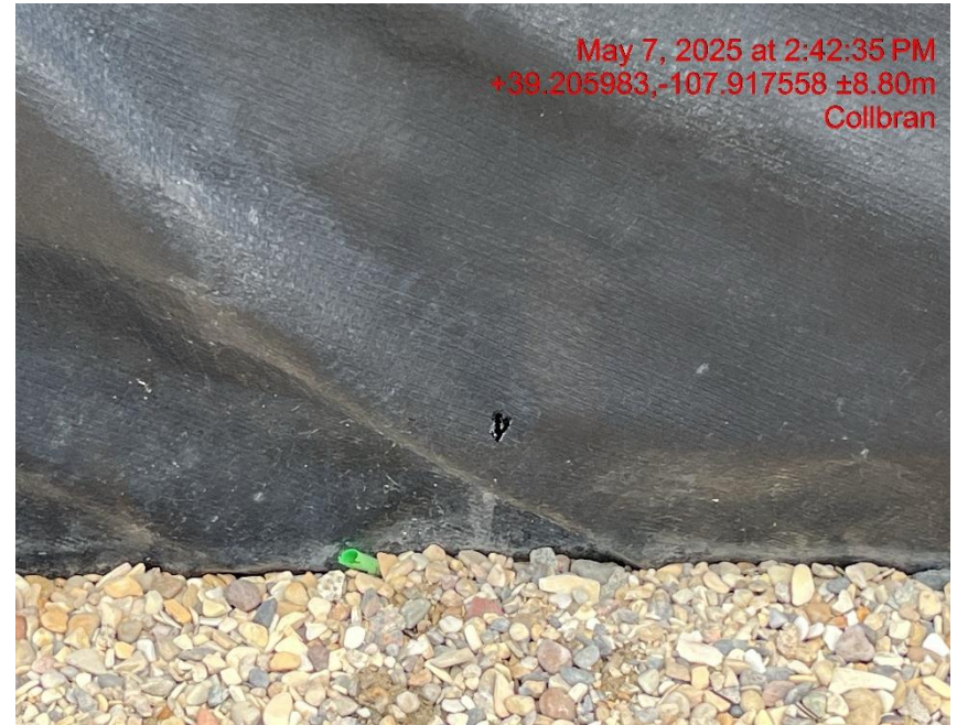
Photo # 7158 Multiple holes in both secondary containments on location liners/liners need maintenance
