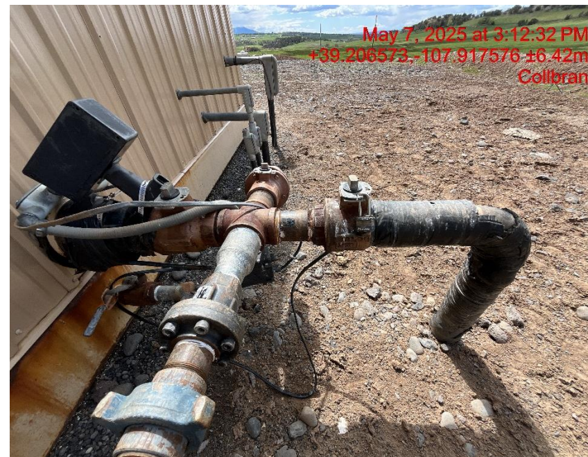
Photo # 7204 Unused flowlines at pump house lack lockout tagout (OOSLAT)
