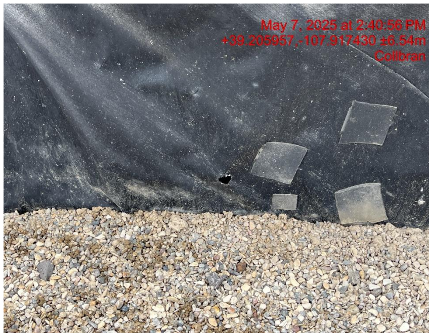
Photo # 7154 Multiple holes in both secondary containments on location liners/liners need maintenance
