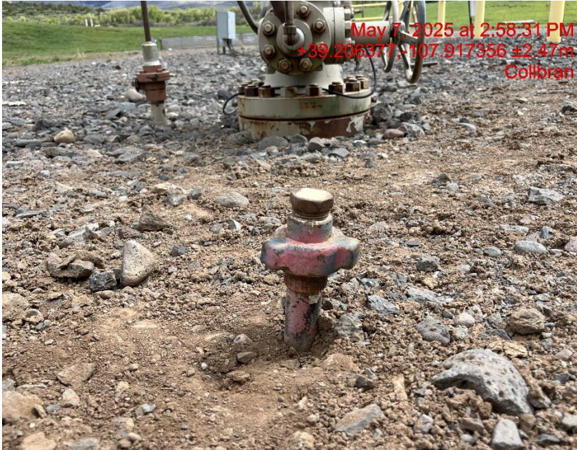
Photo # 7184 Unused flowline near MWR 7-1A wellhead lacks lockout tagout (OOSLAT)
