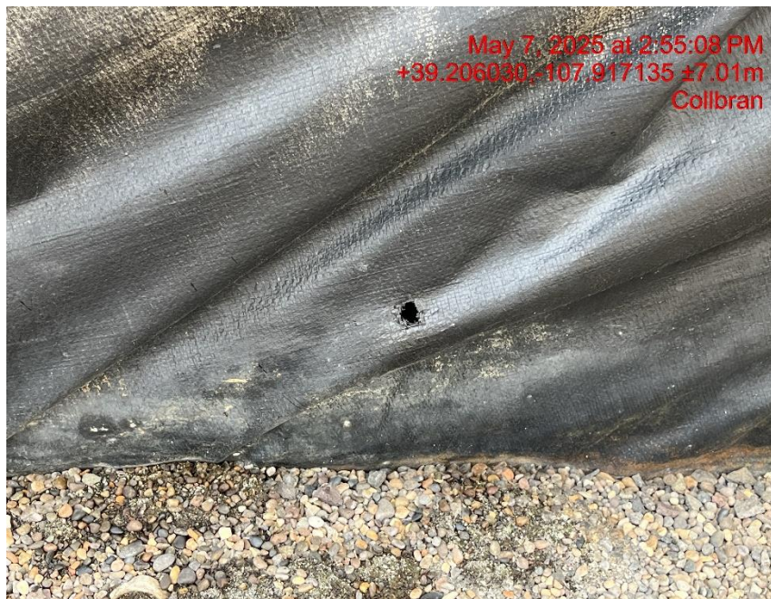
Photo # 7177 Multiple holes in both secondary containments on location liners/liners need maintenance
