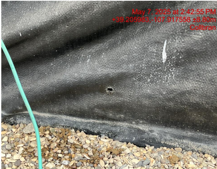
Photo # 7159 Multiple holes in both secondary containments on location liners/liners need maintenance
