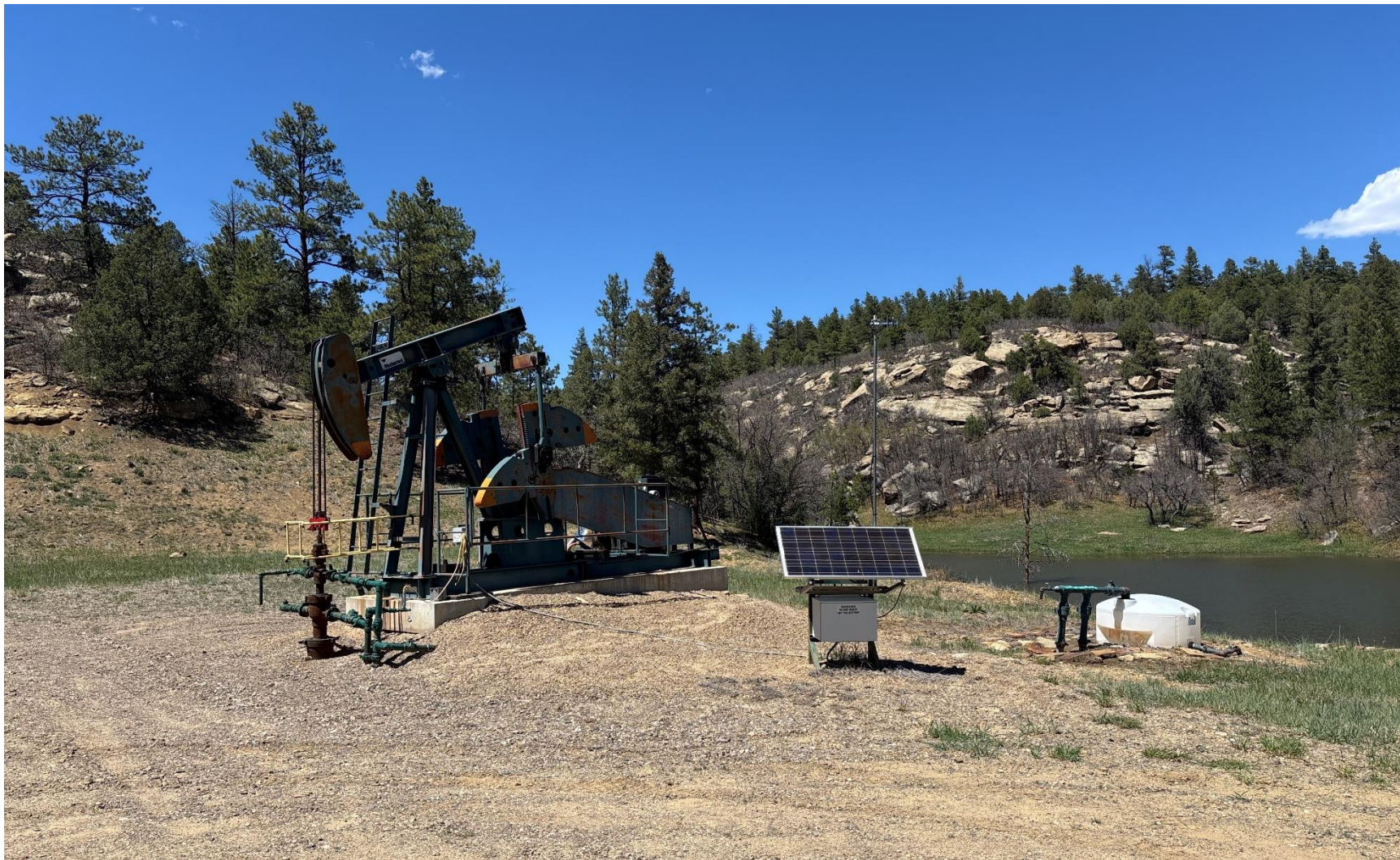
PHOTO 3: WELLHEAD AND EQUIPMENT.
