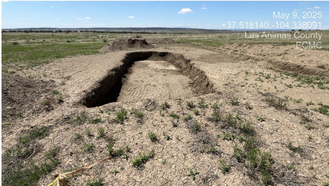
Photo 10. Facing toward the excavation at the southwest corner.
