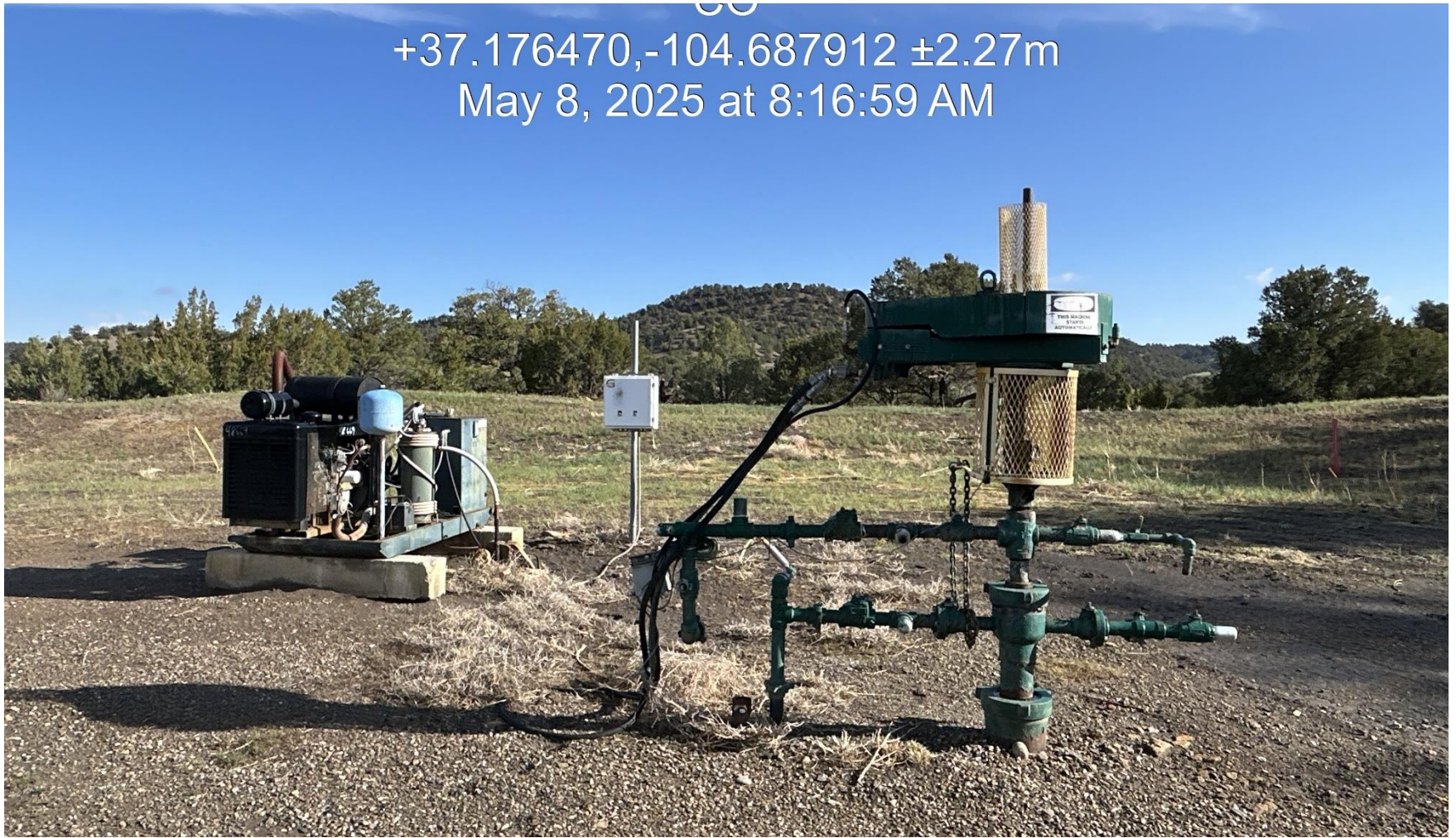
PHOTO 3: WELLHEAD AND EQUIPMENT
