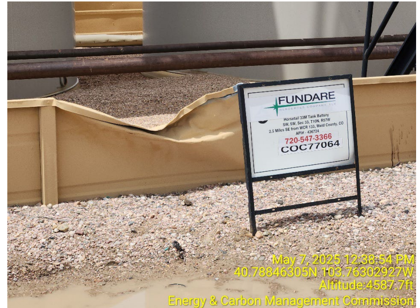
Photo 2 – East Center of Berm is compromised
