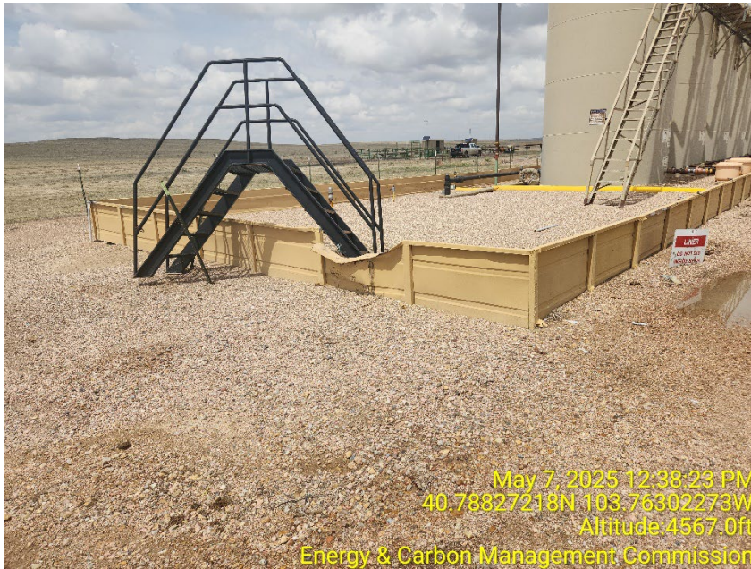
Photo 1 – South end of Berm is compromised
