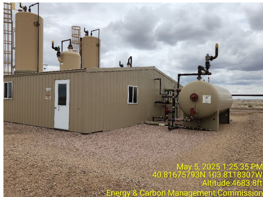
Photo 6 – Heater Treaters
