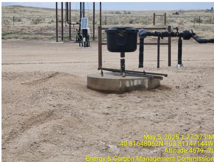
Photo 11 – Signage missing on Compressor Drain Vault
