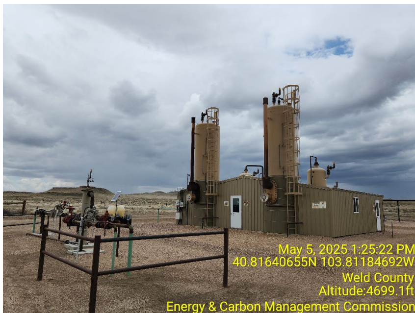
Photo 5 – Heater Treaters
