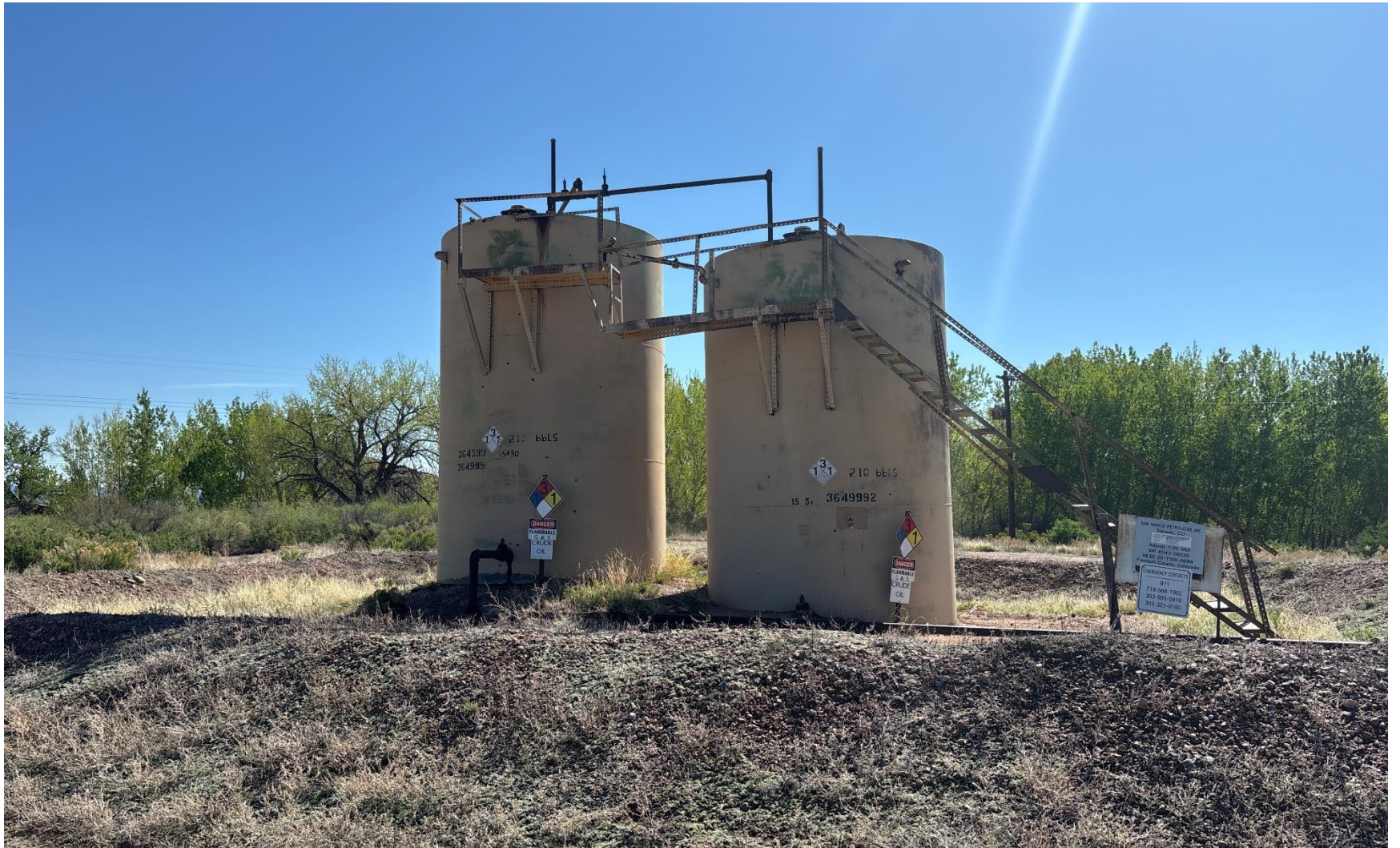
PHOTO 4: WELLHEAD AND EQUIPMENT.
