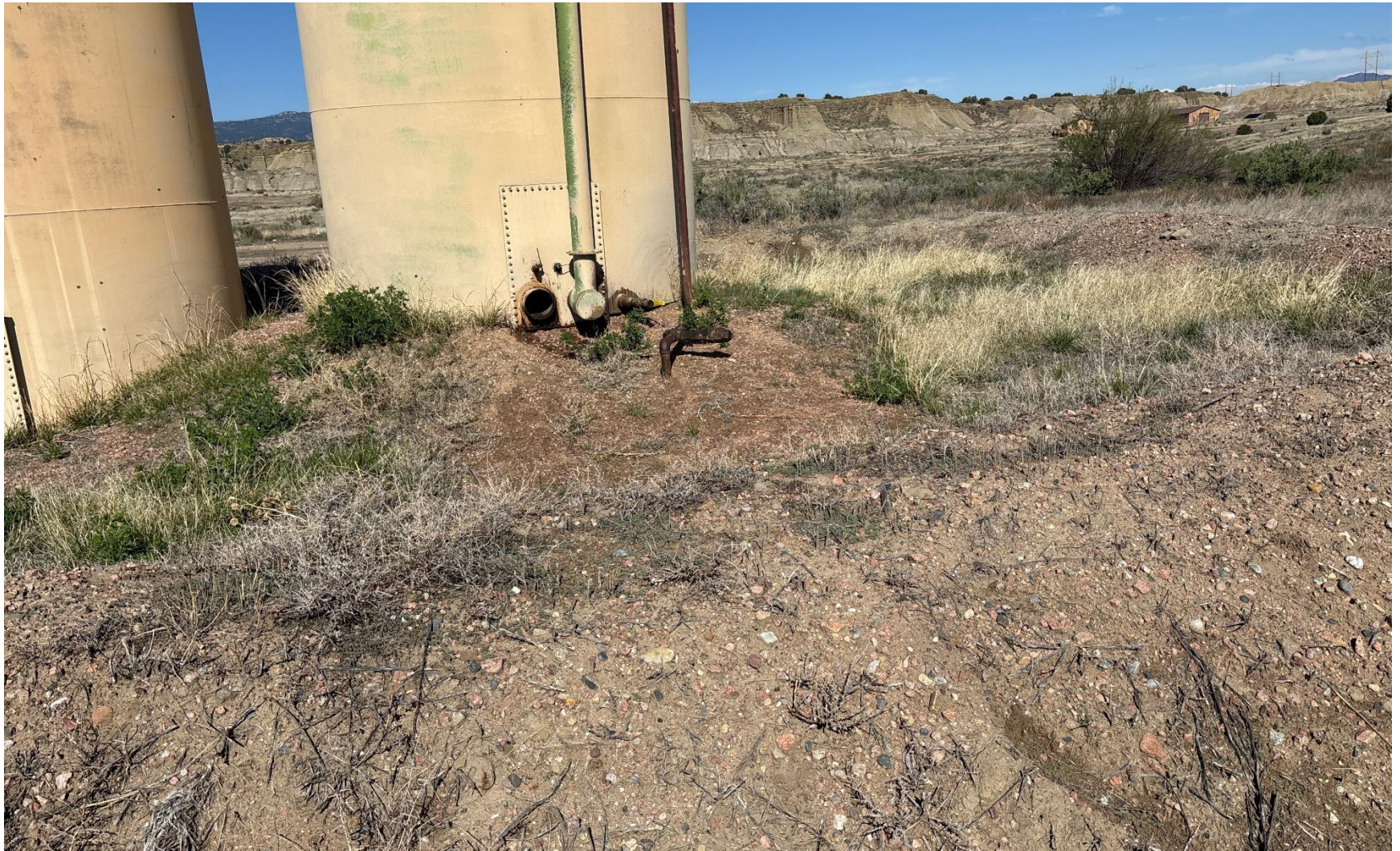
PHOTO 5: WEEDS INSIDE TANK BATTERY BERMS. REMOVE WEEDS INCLUDING ROOT STRUCTURES ON AND INSIDE TANK BATTERY BERMS PER RULE 606. CA DATE 5/21/2025.
