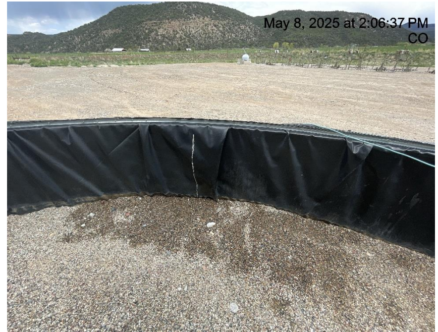
Photo # 40 Staining inside secondary containment
