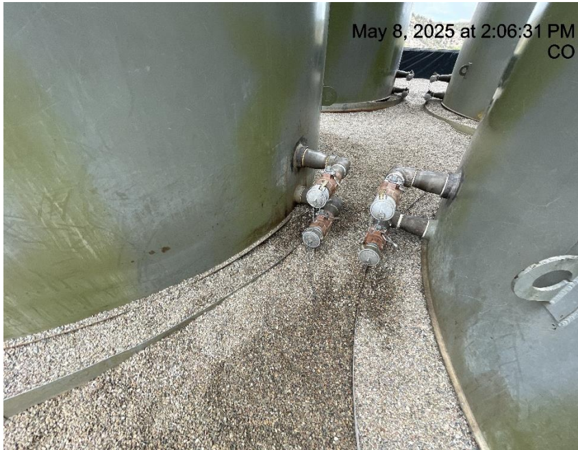
Photo # 39 Staining inside secondary containment
