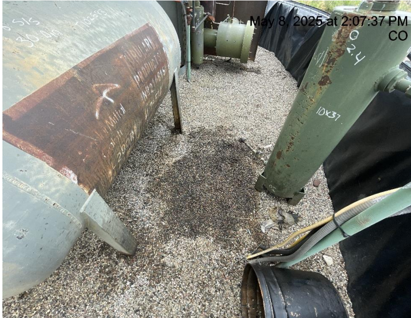
Photo # 41 Staining inside secondary containment
