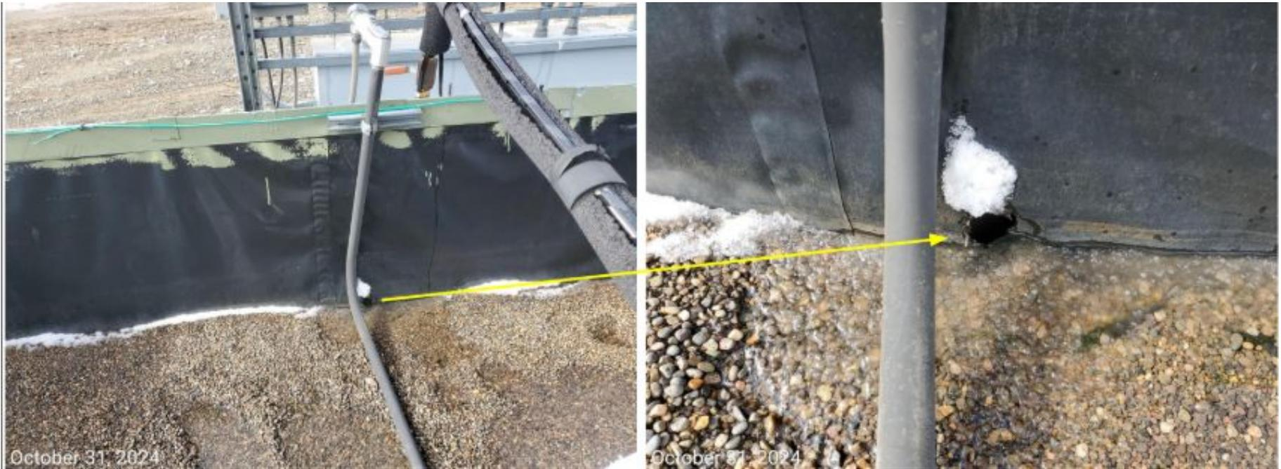
**Photo 1:** Photos taken from the 10/31/2024 inspection. Photos show hole within liner at the tank battery facility documented over multiple inspections.
