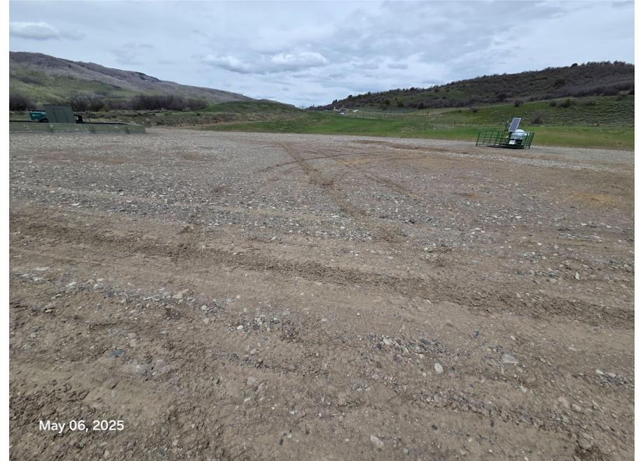
**Photo 3:** BMPs (Gravel/Compaction) to stabilize the working pad surface, and to minimize vehicle tracking/sediment transport is sparse and showing signs of disrepair; tracking/degradation becoming apparent. Maintenance advised.
