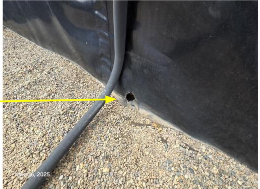
**Photo 2:** Continued from photo 1. Photos dated 5/6/2025. Photos show hole within liner at the tank battery facility has not been repaired; work to ensure that secondary containment remains impervious to contain a spill or release has not been performed, or has been insufficient.
