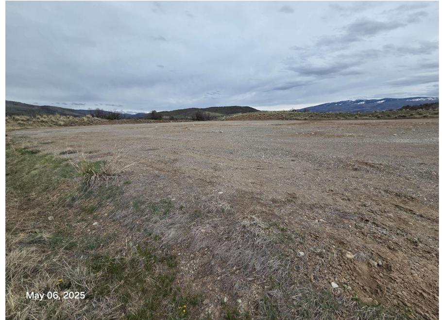
**Photo 1:** Photos 1-3 taken from the south end of the working pad surface. Photos provide an overview of the Location from west, northwest, northeast, southeast to southwest. Location and access road are subject to 1004 Final reclamation requirements including, but not limited to removal of gravel, compaction alleviation, recontouring/regrading, replacement of topsoil and revegetation activities by 7/9/2025.
