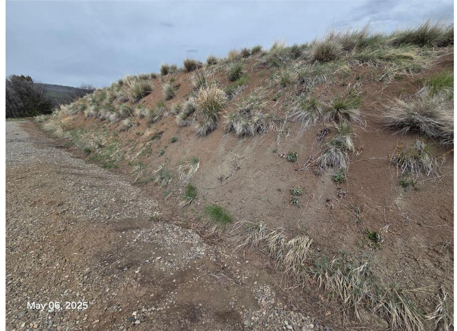
**Photo 4:** Photo taken from the Topsoil stockpile on the northwest end of the Location. BMPs to stabilize soils remain missing or insufficient; soils are bare and at risk to wind and water erosion.
