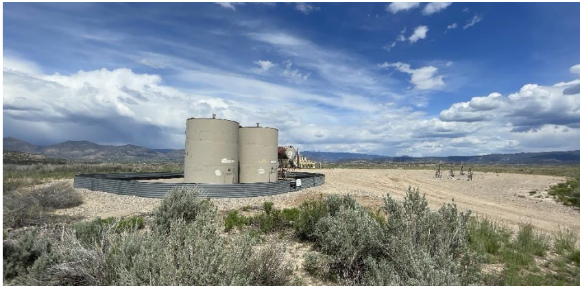
South West corner of location.
