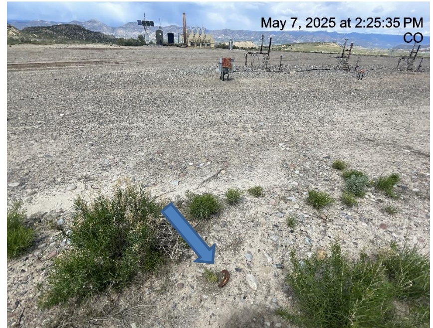
Photo # 9461 Same unmarked deadman
