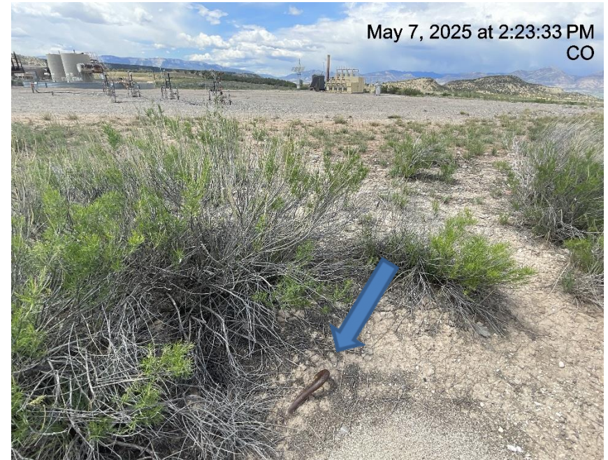
Photo # 9459 Same unmarked deadman from a different angle
