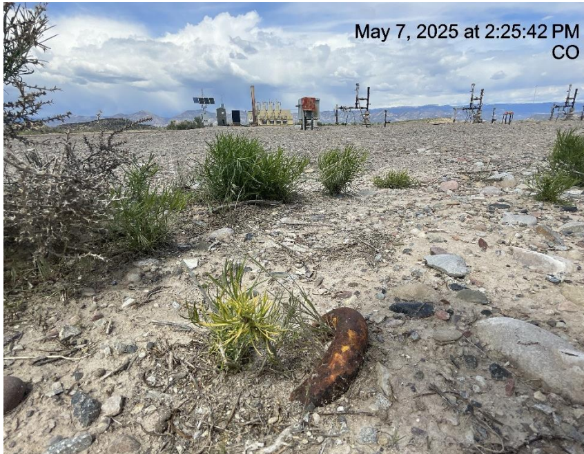
Photo # 9462 Same unmarked deadman from a different angle
