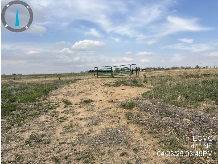
Photo 5. Photo taken of the access road, at the entrance to the location, facing Northeast. Photo illustrates that vegetation establishment does not meet Rule 1004 reclamation standards.
