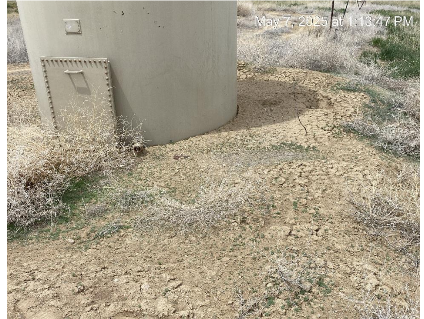
Inadequate tank berm bordering wetland drainage.
