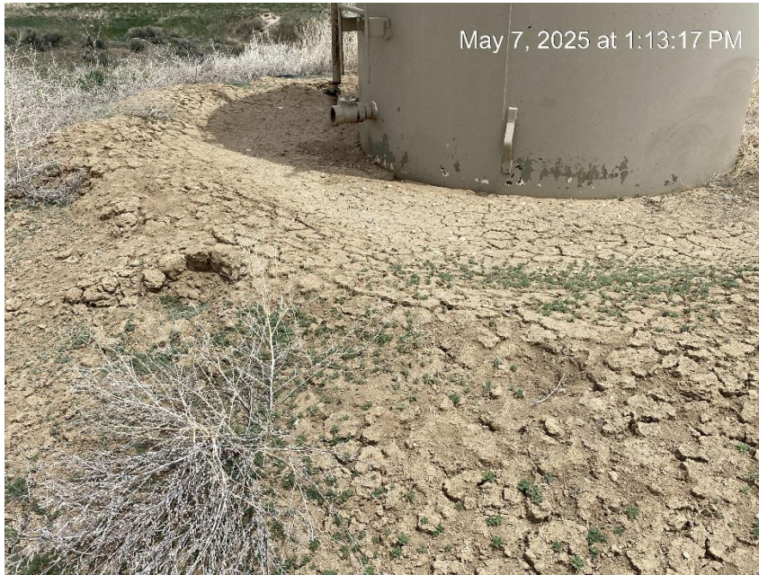
Inadequate tank berm. Borders wetland area.
