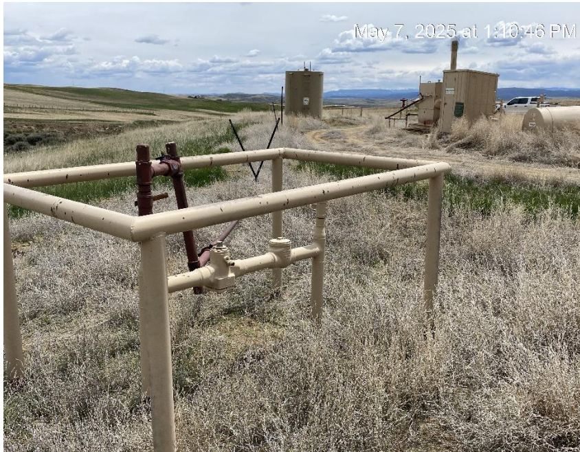
Blow down line. Broken connection at tank
