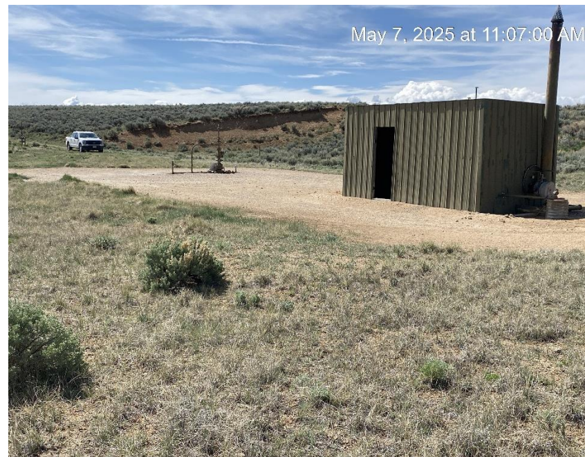
Location from North corner
