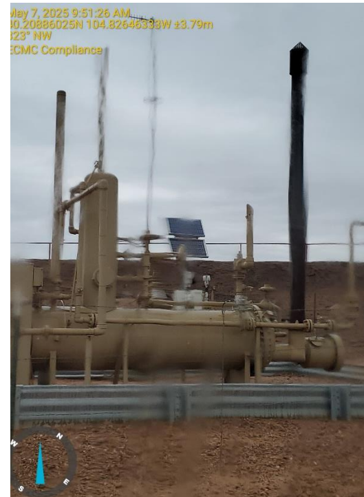
Heated Horizontal Separator
